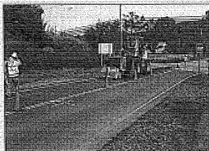
Removing AC with Zipper
