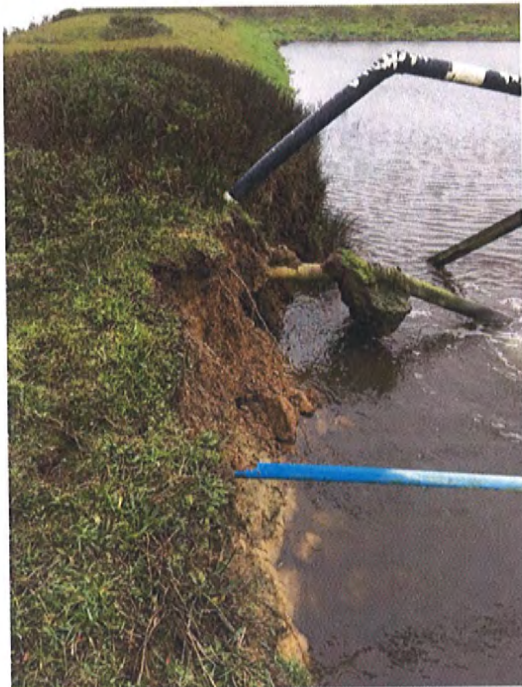
Ocean Marin Treatment Pond 1/10 Before temporary repairs
