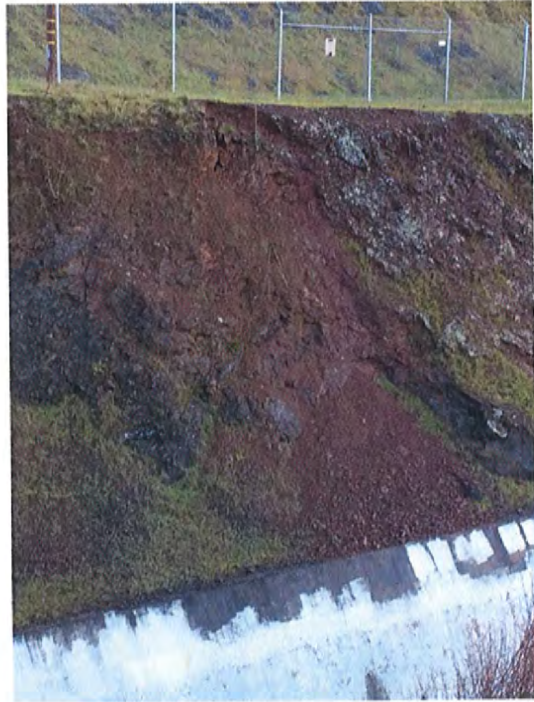
Spillway erosion
