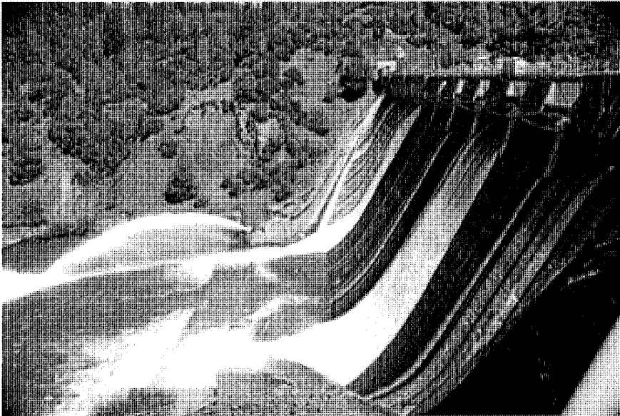
The 130ft-tall Scott Dam on the Eel River, which stores water for year-round power production and irrigation. Photo Courtesy Potter Valley Irrigation District
