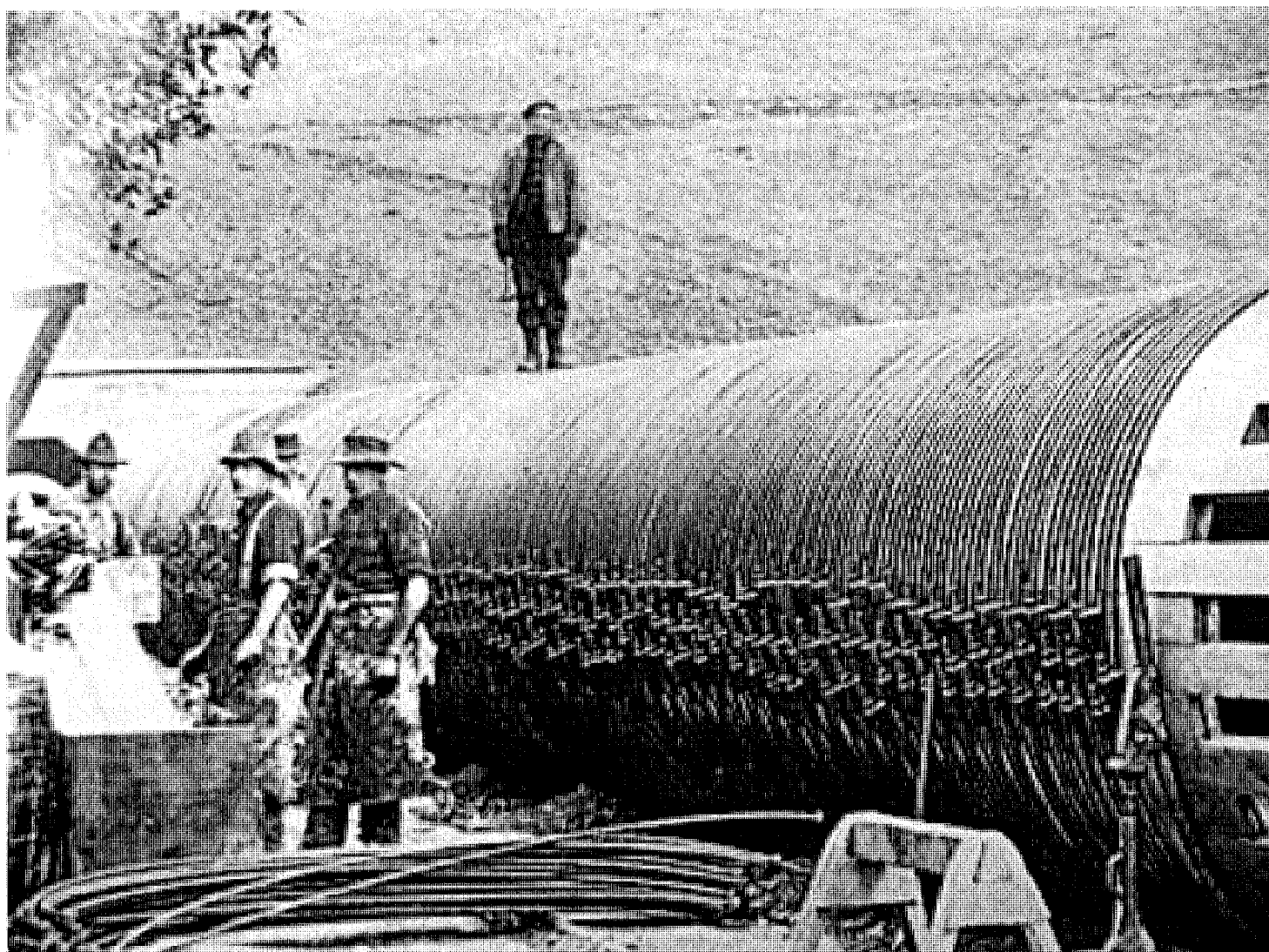
The original sluice serving the Potter Valley powerhouse, shown here, was built of redwood and completed in 1908. (Photo Courtesy Potter Valley Irrigation District)
