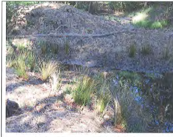
Spoils area above double culverts
