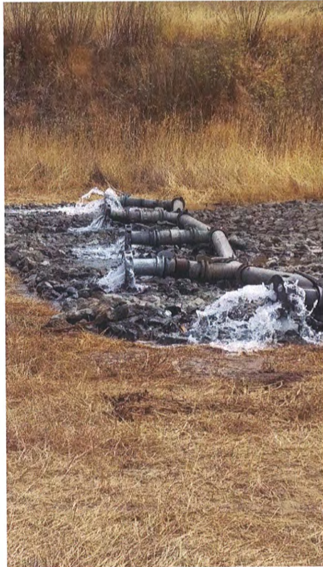
Discharge of Flushing Water in Majauskas Field (8/19/15) (See Photo Location # 5 on Slide 2)
