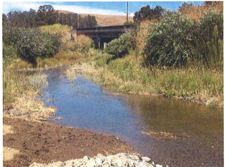
Flushing Discharge Into San Antonio Creek (8/21/15) (See Photo Location # 6 on Slide 2)
