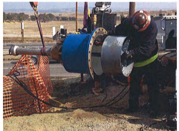
11/11/2013 Removing the Coupon from Hot Tap Machine at One of the Line Stop Locations
