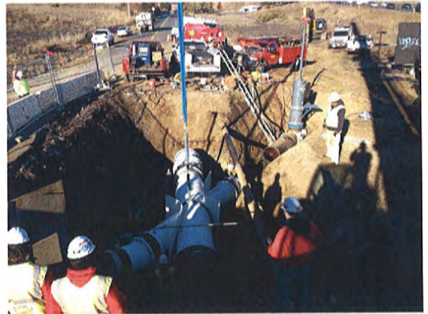
12/10/2013 Setting the Cut-In Pipe Spool at the North End Connection for W-2 Pipeline Segment
