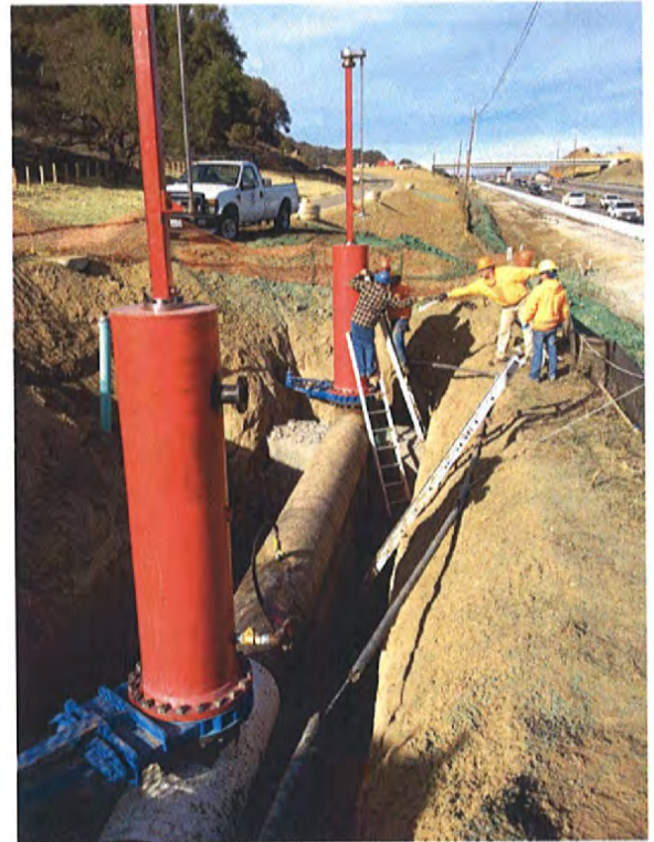
12/6/2013 View of Two Installed Line Stops at the South End of the W-2 Pipeline Segment
