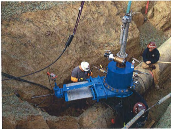
11/11/2013 Installing the Temporary Knife Gate and Hot Tap Machine at One of the Line Stops
