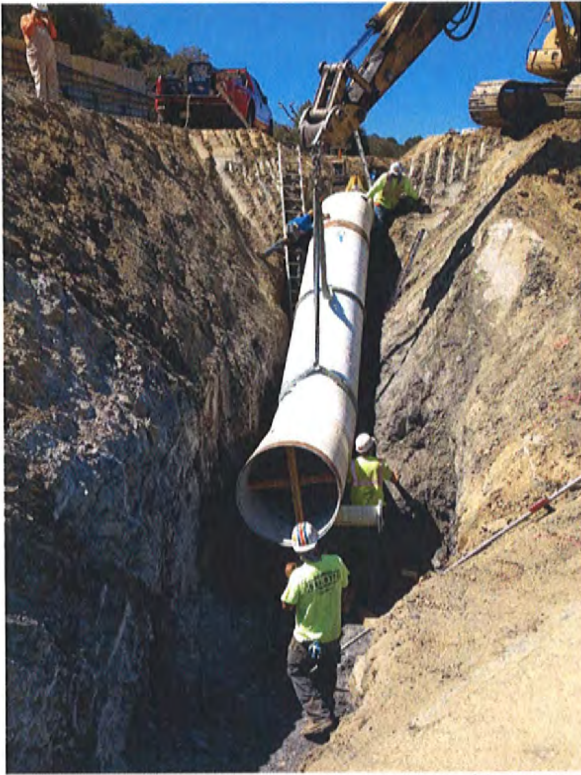
9/1/2013 Installing Pipe w/a Slope of .595 Located North of the Over Pass
