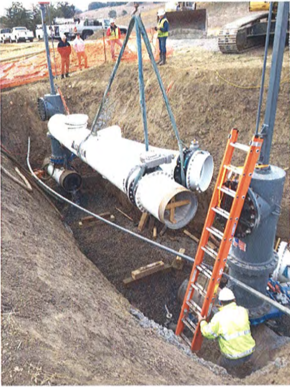
1/8/2014 Setting the Cut-In Pipe Spool at the South End Connection for W-1 Pipeline Segment
