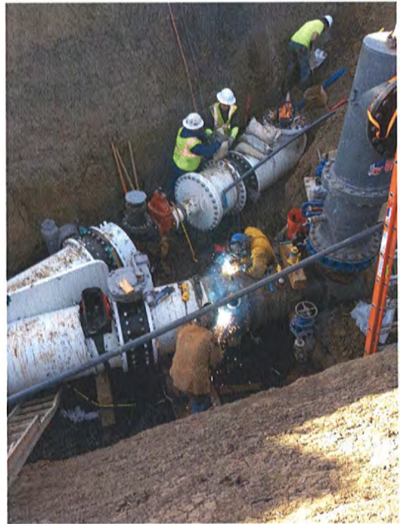
1/8/2014 Setting the Cut-In Pipe Spool at the North End Connection for W-1 Pipeline Segment
