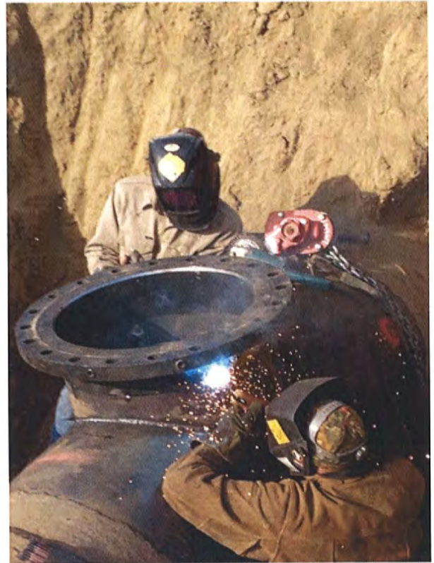
11/6/2013 Welding Flanged Outlet for One of the Line Stops
