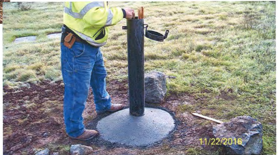
Rehabilitated Piezo Well Head
