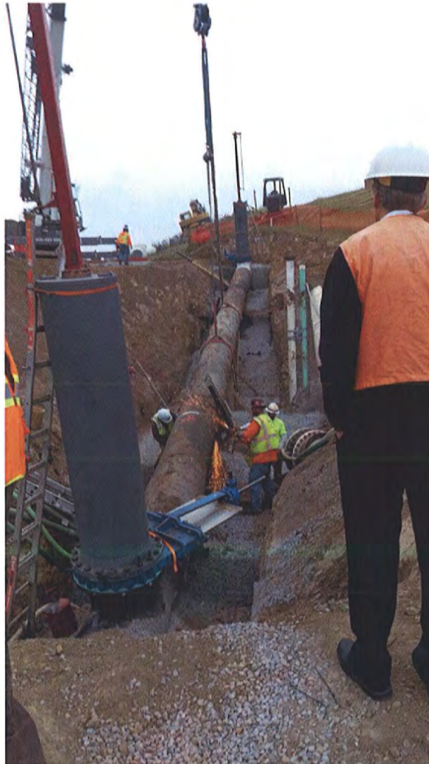
Existing Pipe at Middle Connection (See Photo Location #13 on Slide 2)
