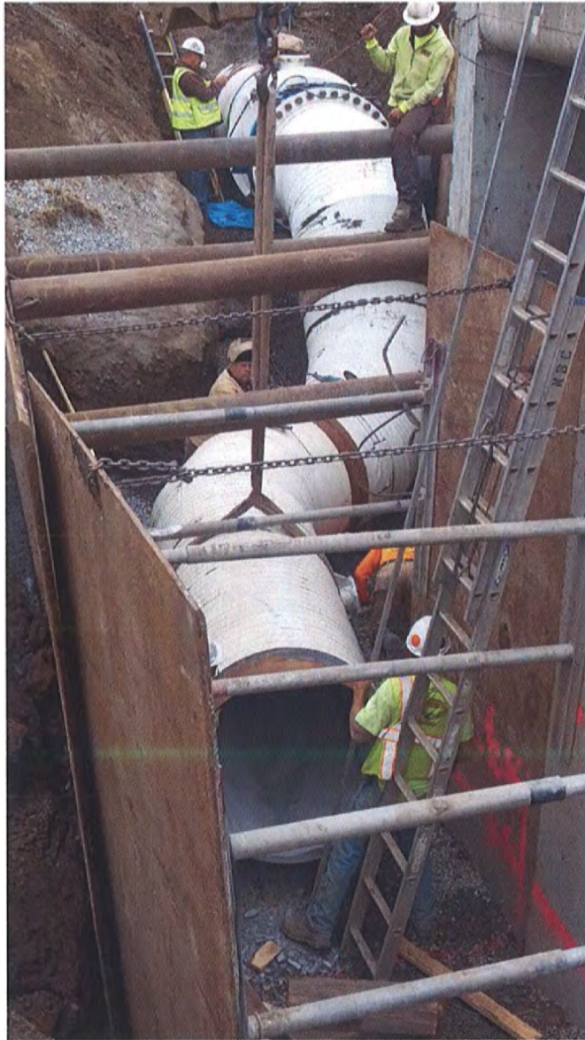
Pipe Installation at Box Culvert (See Photo Location #15 on Slide 2)
