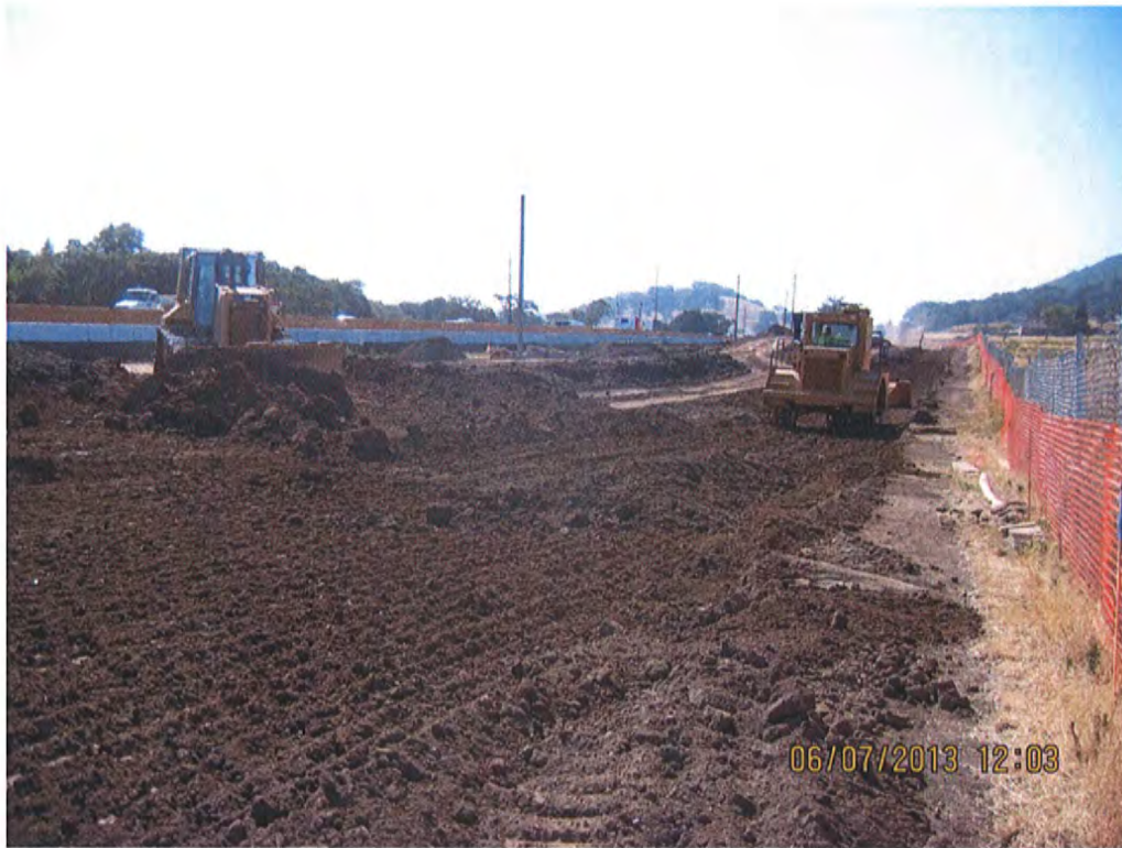
Backfill/Compaction Operation for the Trench Zone
