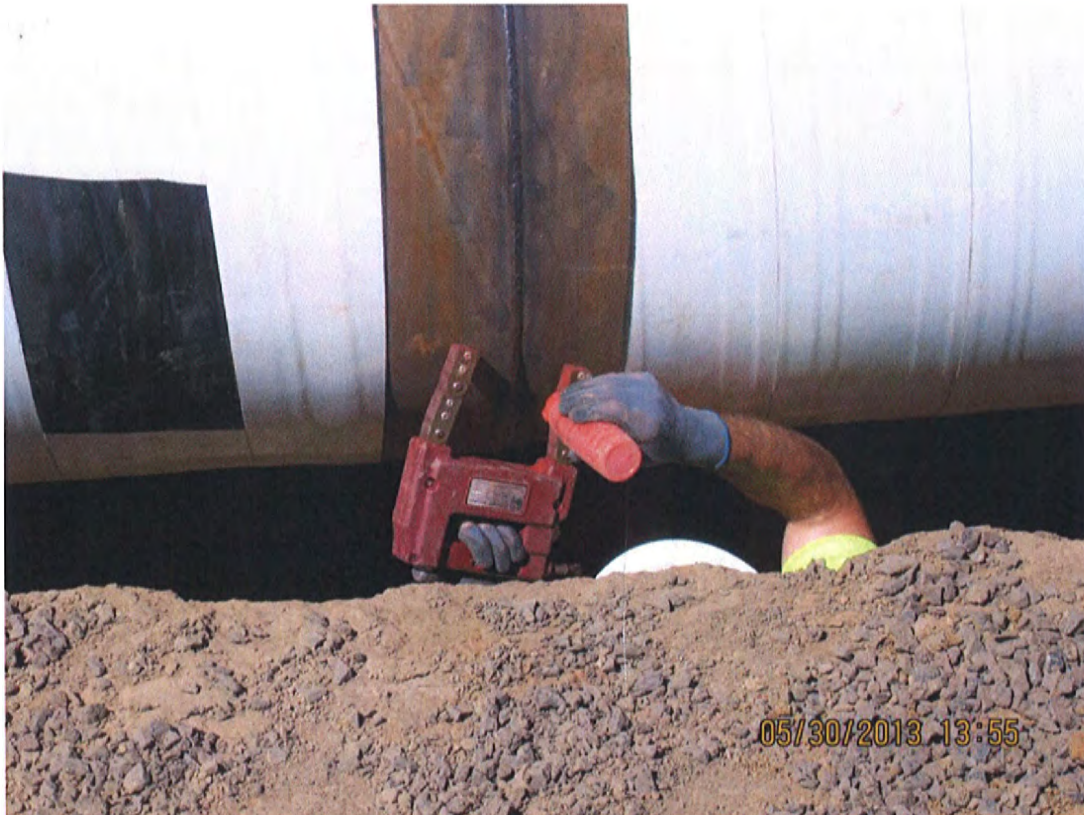
Magnetic Particle Testing of the Lap Welded Pipe Joint
