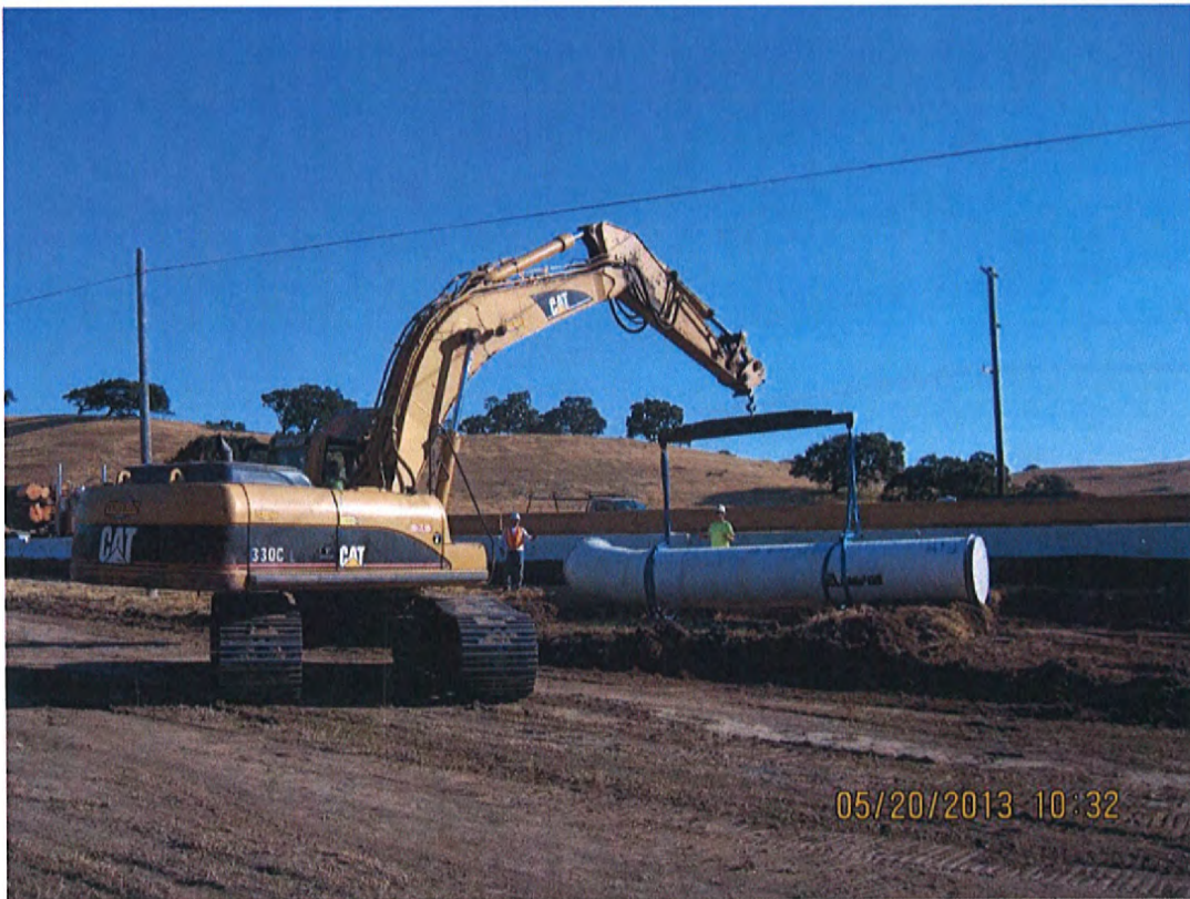
Staging 42" WSP on Earth Berms, Note Nylon Straps
