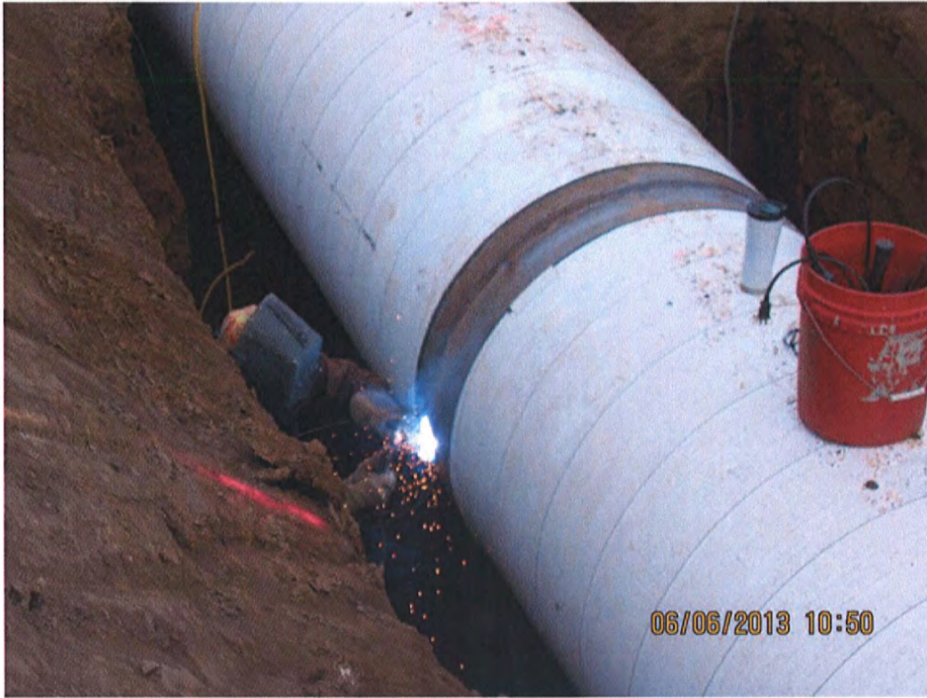
Lap Welding 42" Pipe Joint
