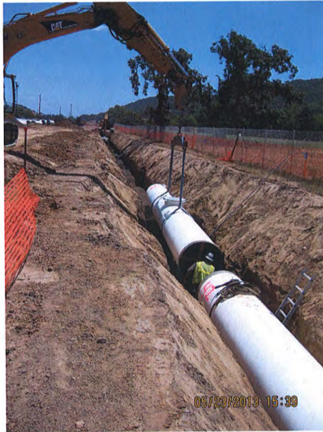
Installing a Piece of 42" WSP that Contains a Manway
