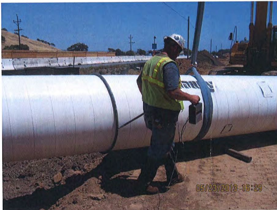
Spark Testing the Tape Wrapped Coating Using 36,000 Volts
