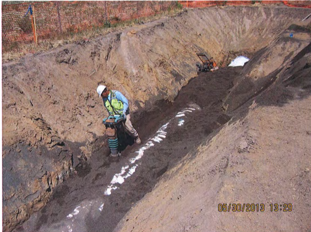
Compacting the Import Sand Pipe Zone
