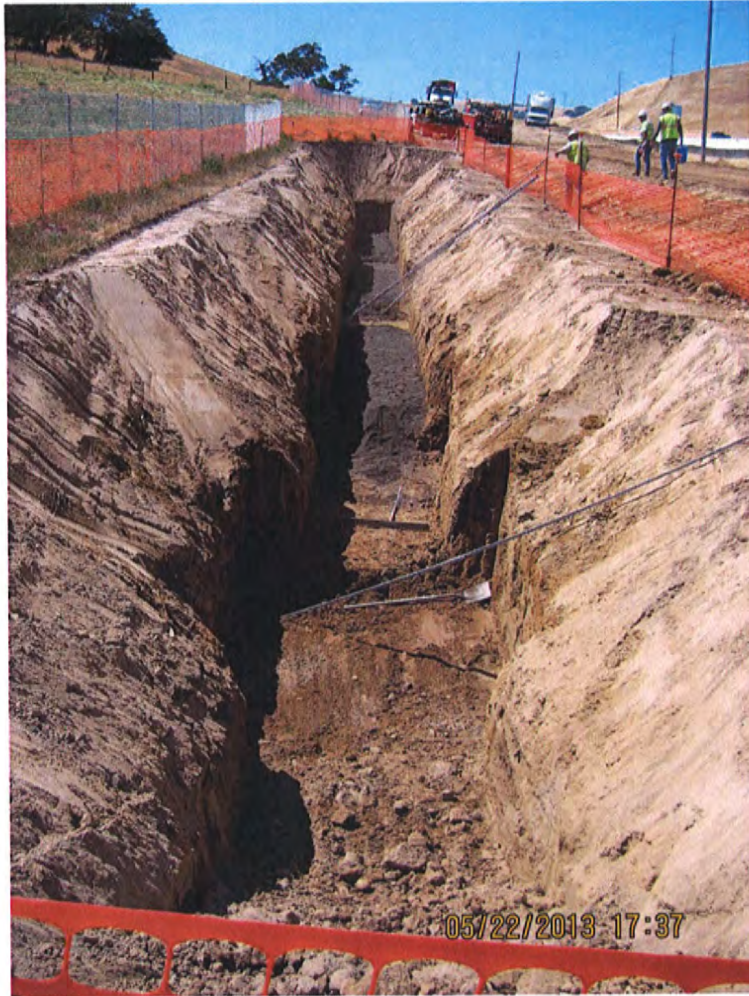
Prepared Excavated Trench w/6" Sand Bedding
