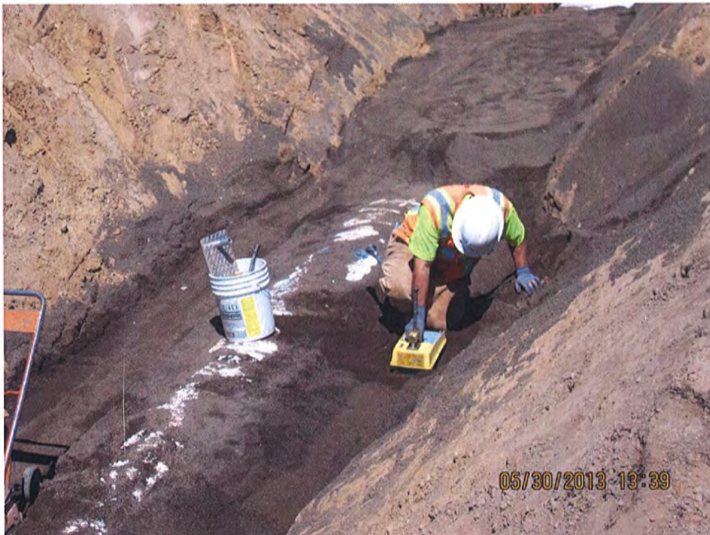
Testing the Imported Sand Compacted Pipe Zone
