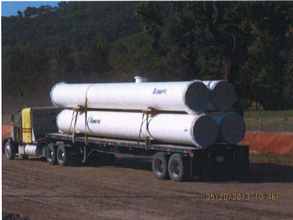
Pipe Delivery From Ameron's Plant in Tracy, CA
