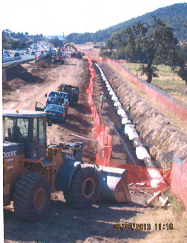
First Section of Installed Pipeline
