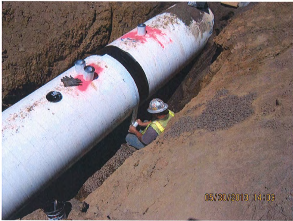
Tape Wrapping a Field Weld Pipe Joint
