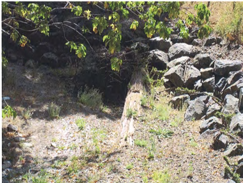
Figure 5. Log vane after winter flows showing scour and aggradation of channel to create channel complexity, looking downstream (PCI June 2013).
