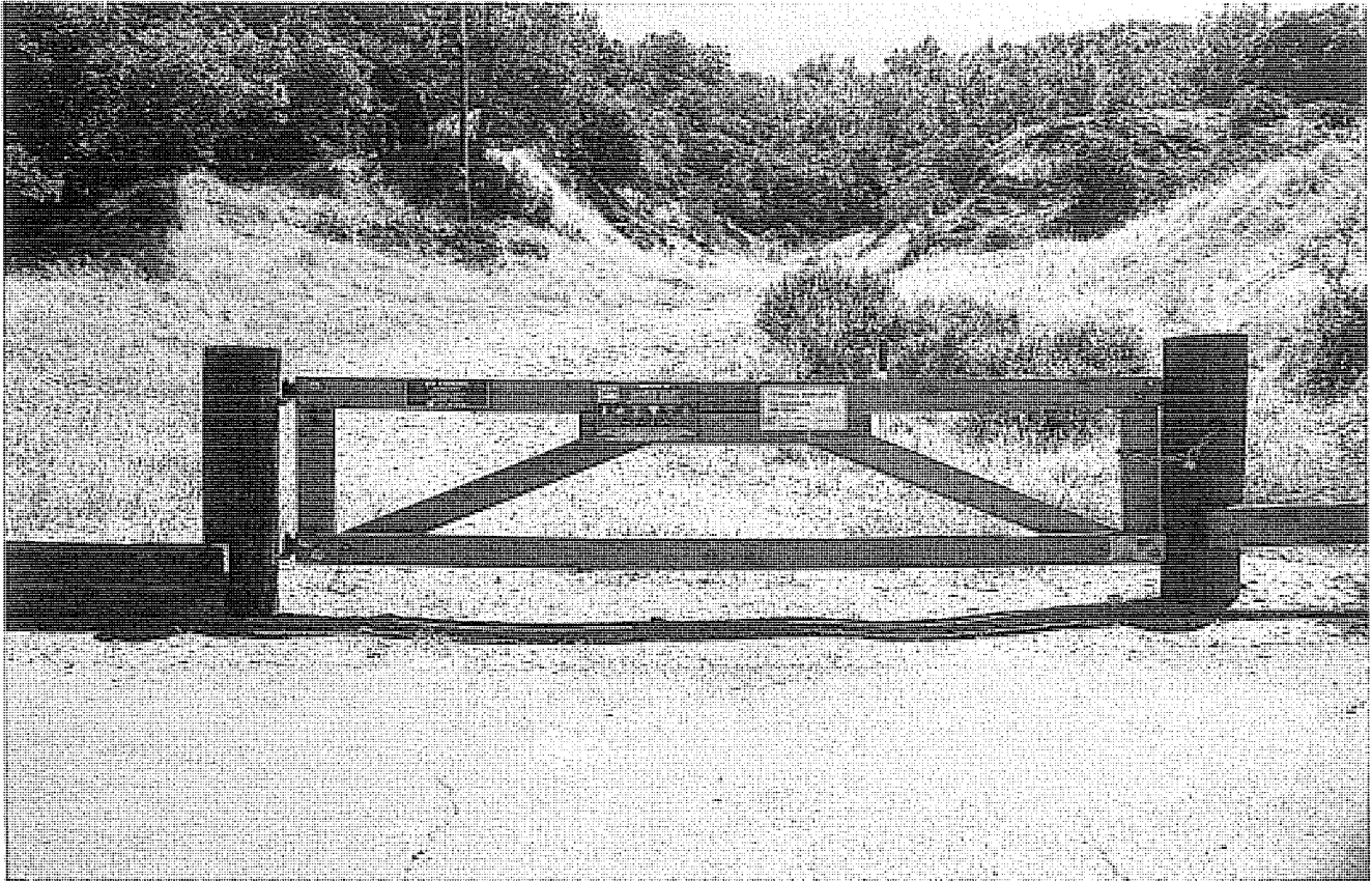
Lower section of access and utility route and the gate at the top of Winged Foot Drive
