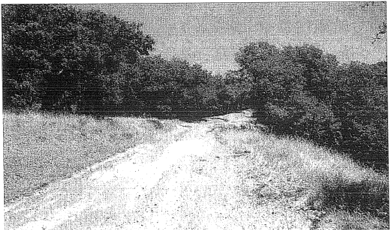
Upper section of access and utility route
