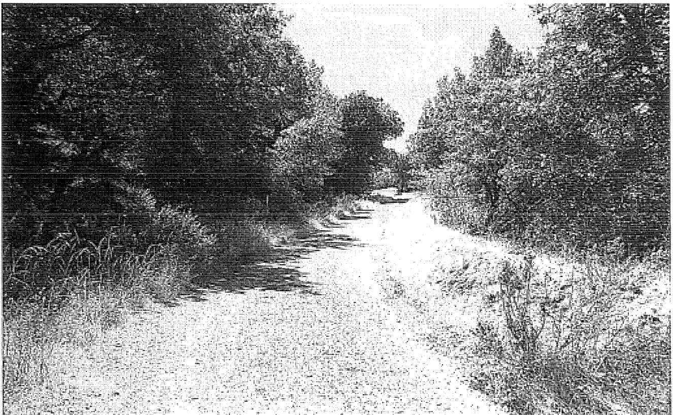
Lower section of access and utility route looking up to midway section
