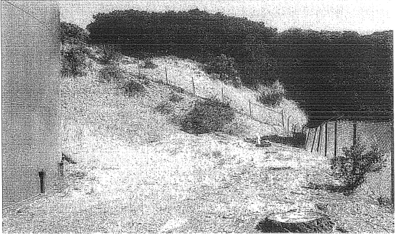
Looking east to equipment location at rear of tank
