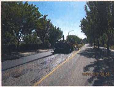
Asphalt Grind and Overlay on Main Gate Rd
