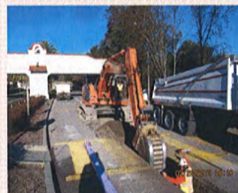
Excavation on Main Gate Rd
