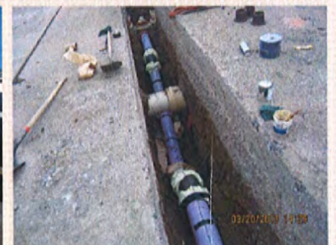
45 deg bends underneath (E) main
