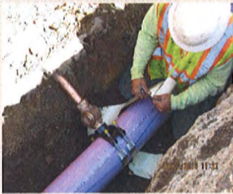
O-Line Service Lateral Installation
