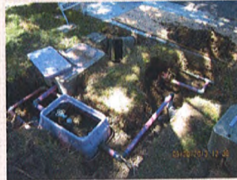
Irrigation Retrofits on Hamilton Pkwy
