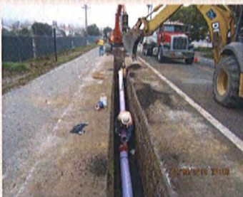
Pipe Installation on State Access Rd
