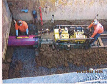
Jack & Bore under RR Tracks
