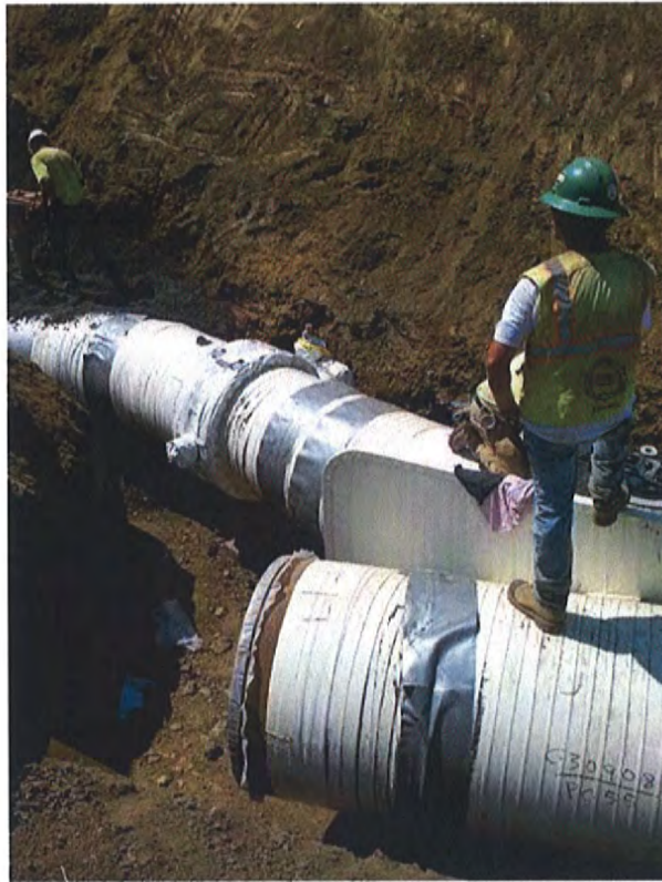
Installation of wye for connection point north of Korean Church property (6)
