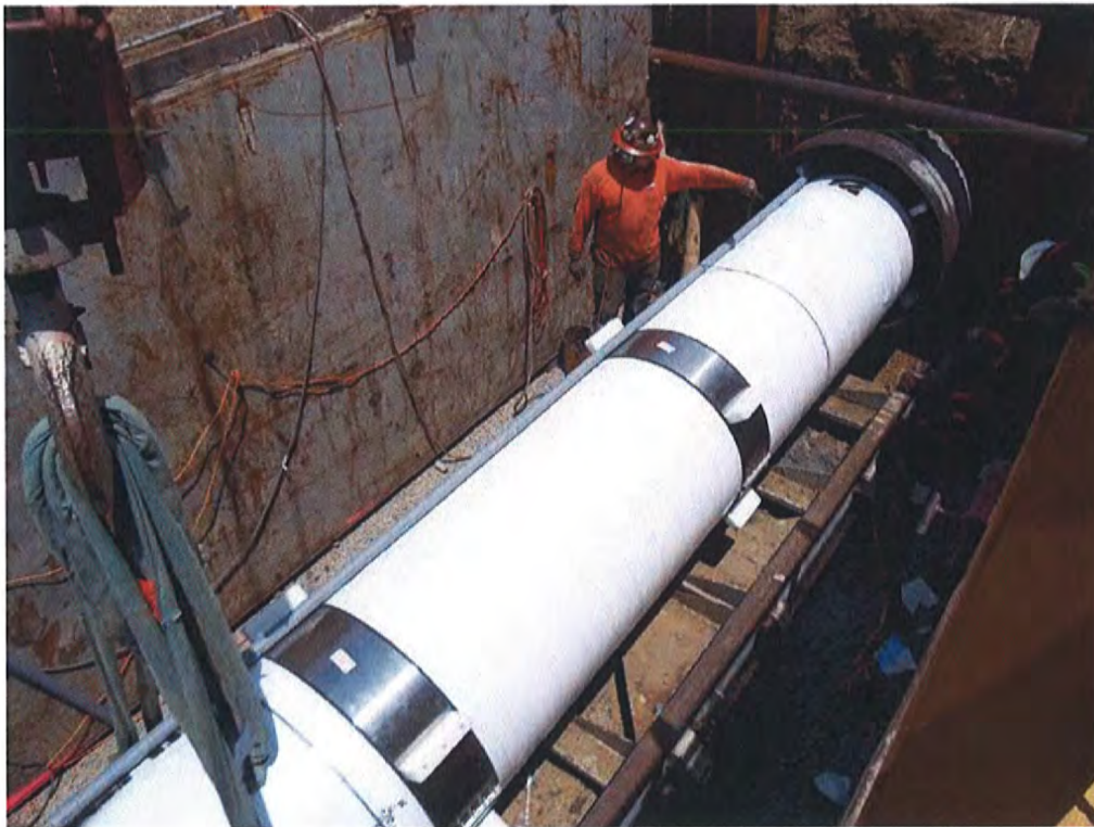
Installing Carrier Pipe in casing at North Highway 101 Crossing (2)
