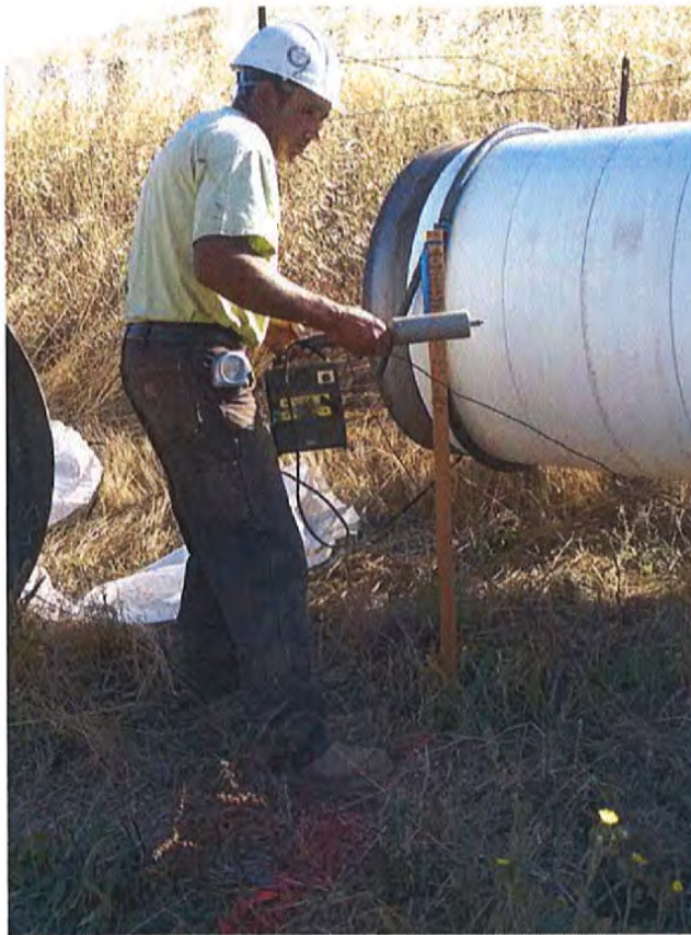
Testing of Tape Wrap Prior to Pipe Installation (3)
