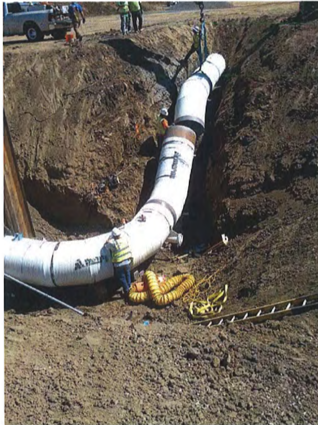
Pipe installation out of jacking pit crossing Hwy 101 on Tognalda Property (9)
