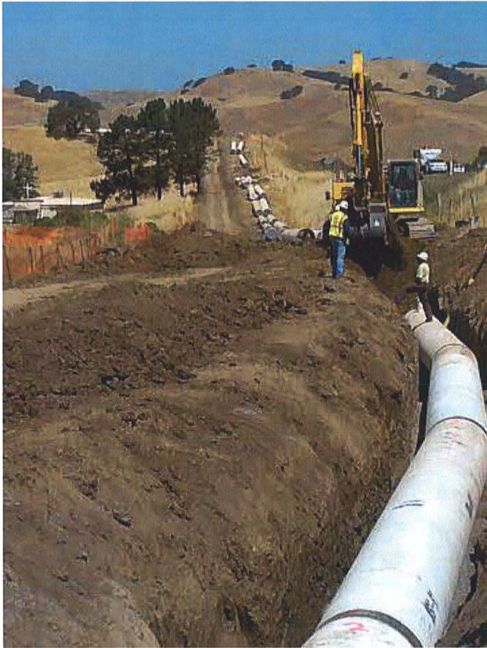
Pipe Installation in Reach D (5)
