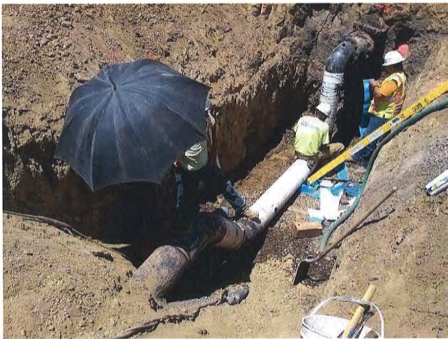
Work on 10 inch Drop (4)
