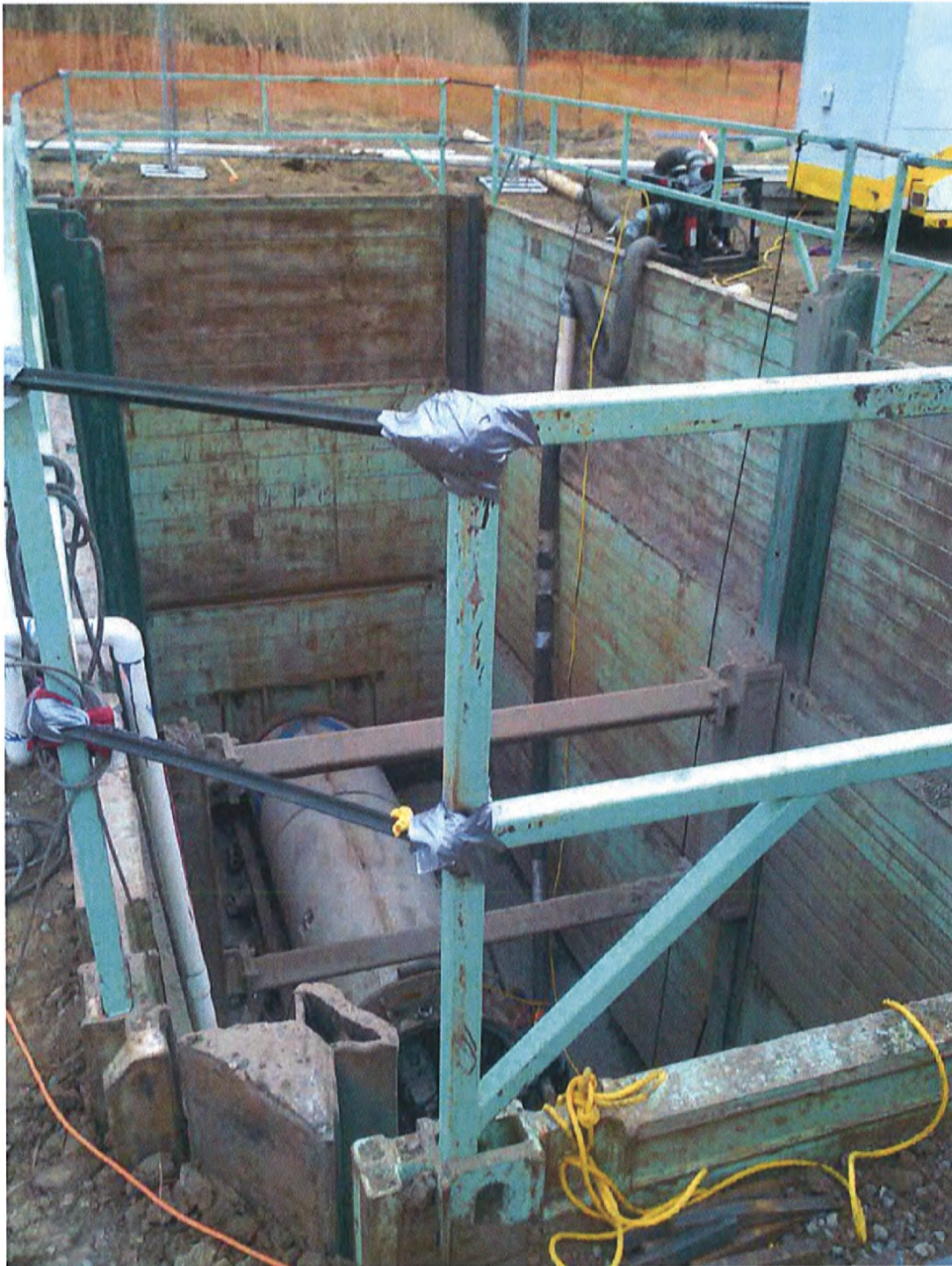
Jacking pit on Tognalda Property for crossing of San Antonio Creek (10)
