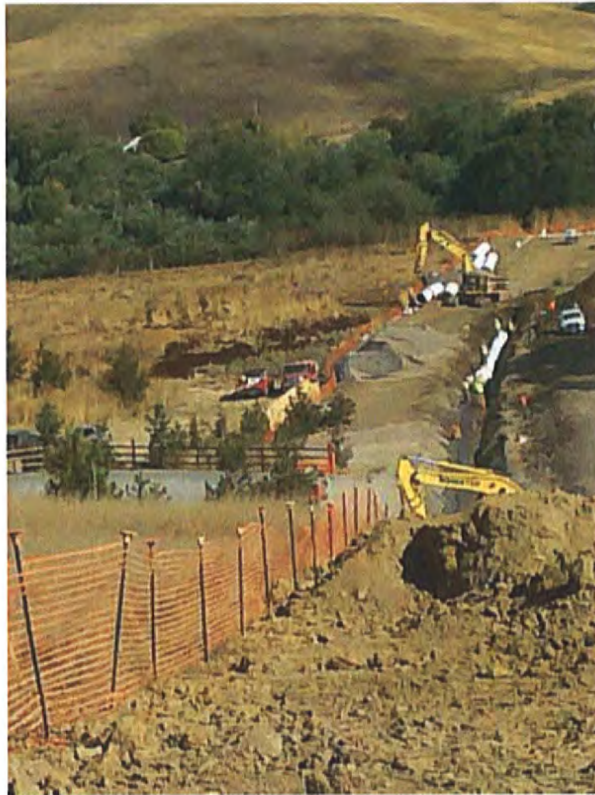
Pipe installation looking north from hill behind the Korean Church (8)
