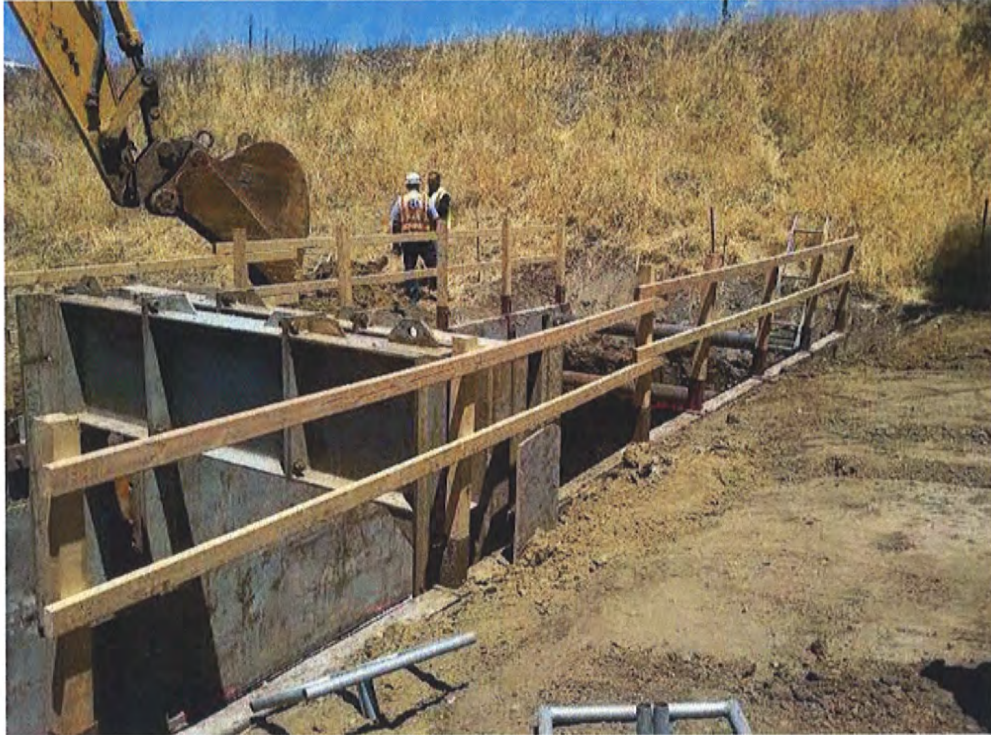
Jacking Pit for North Highway 101 Crossing (1)
