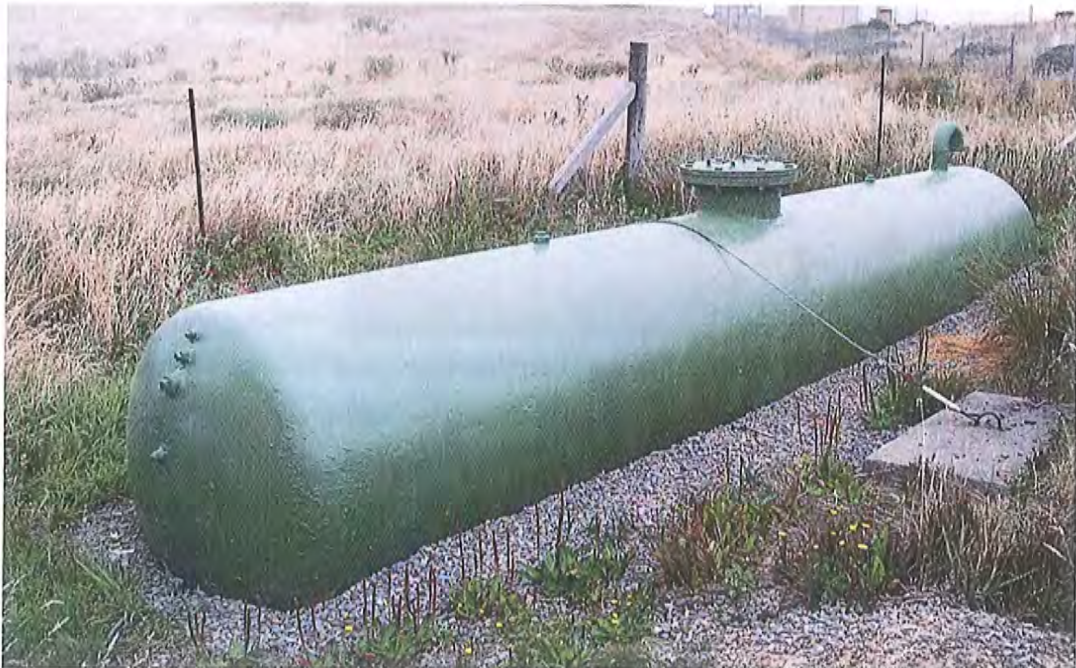
Oceana Marin Dosing Tank Re-Stored and Re-Coated
