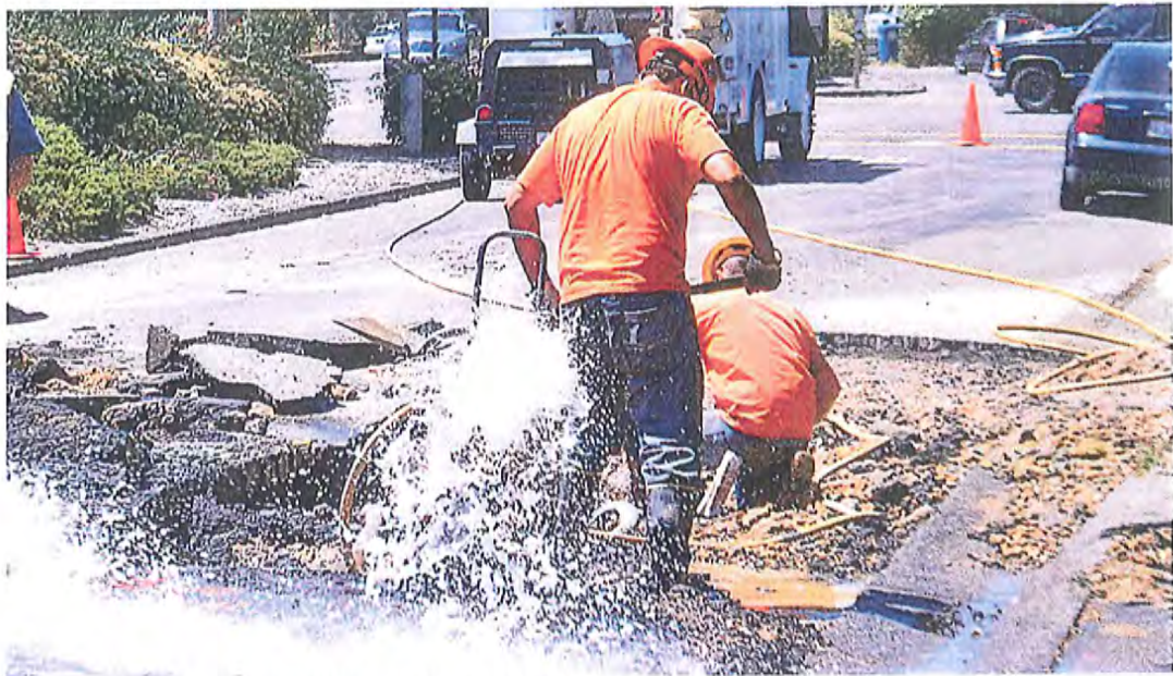
NMWD crew fixing a 12" cast iron main break on Sunset Parkway
