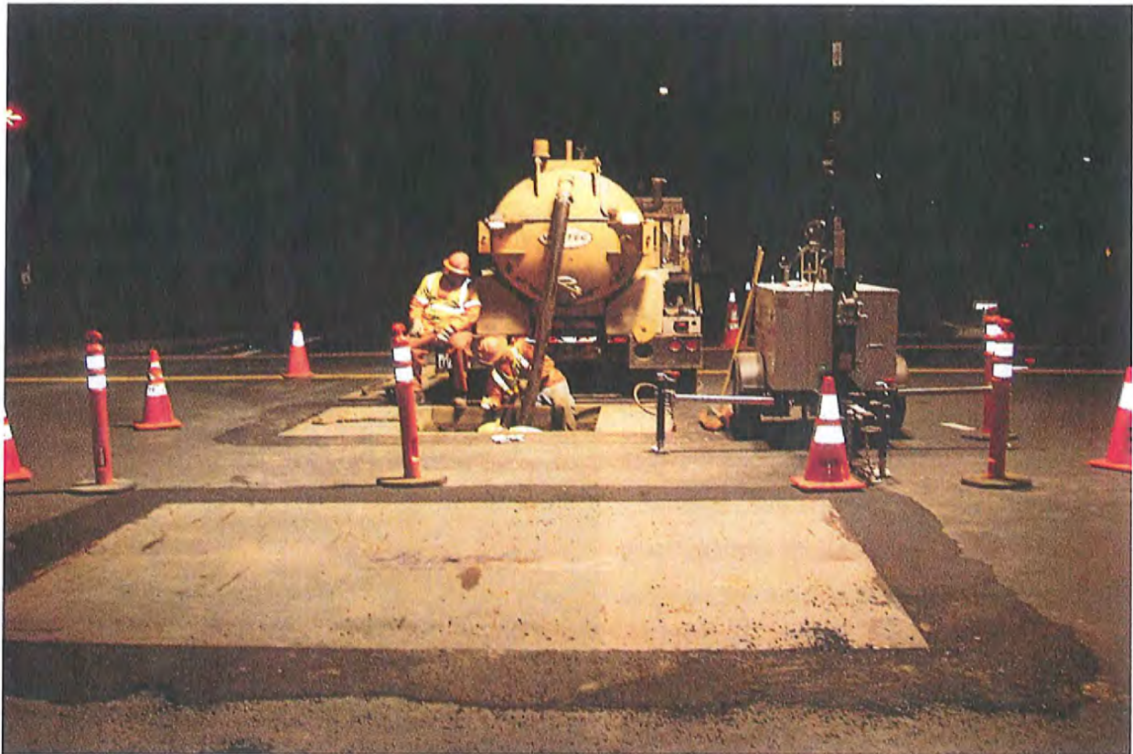
South Novato Main Break Repair
