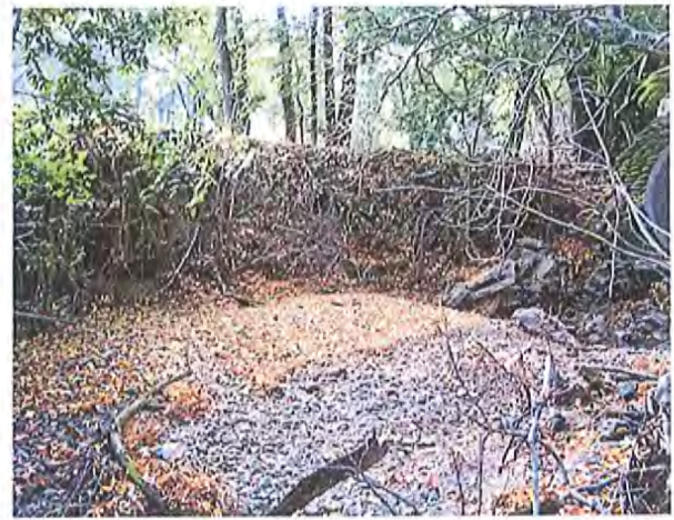
Leveroni Creek Bank Repair
