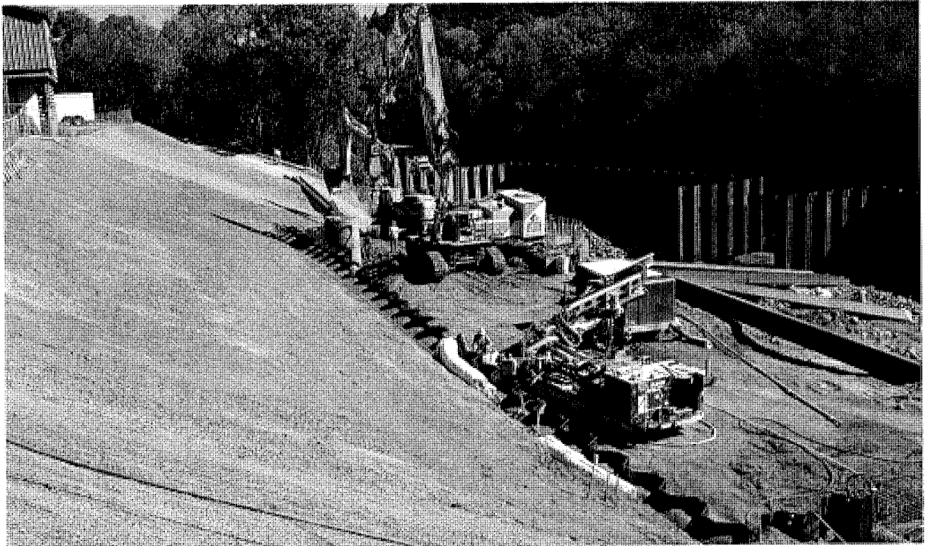
Mirabel Fish Passage Improvement Project, September 2014
