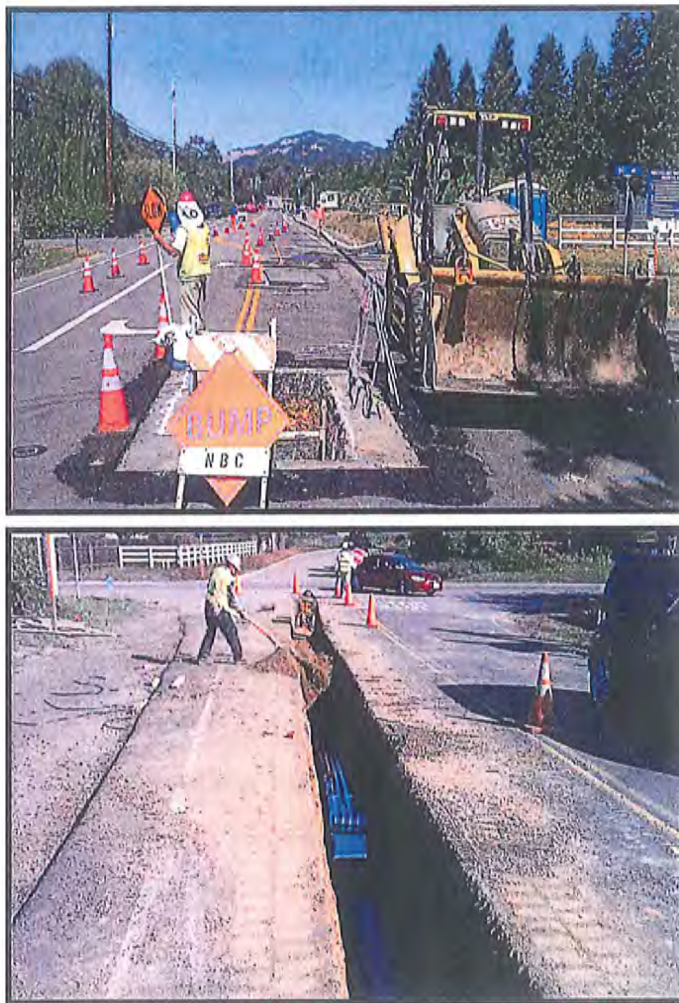
Recycled Water Segment 1 & 3
