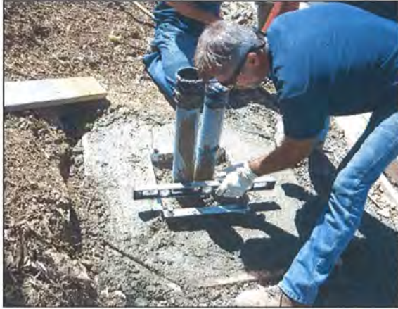
Bolling Circle RWF Pump Station
