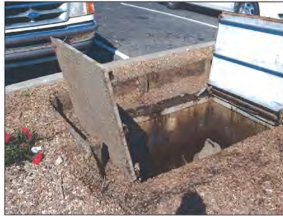
Fire Service Vault Removal on Rowland Blvd.
