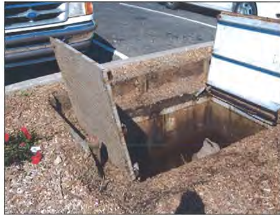
Fire Service Vault Removal on Rowland Blvd.
