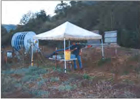
Gallagher Well Test Operation
