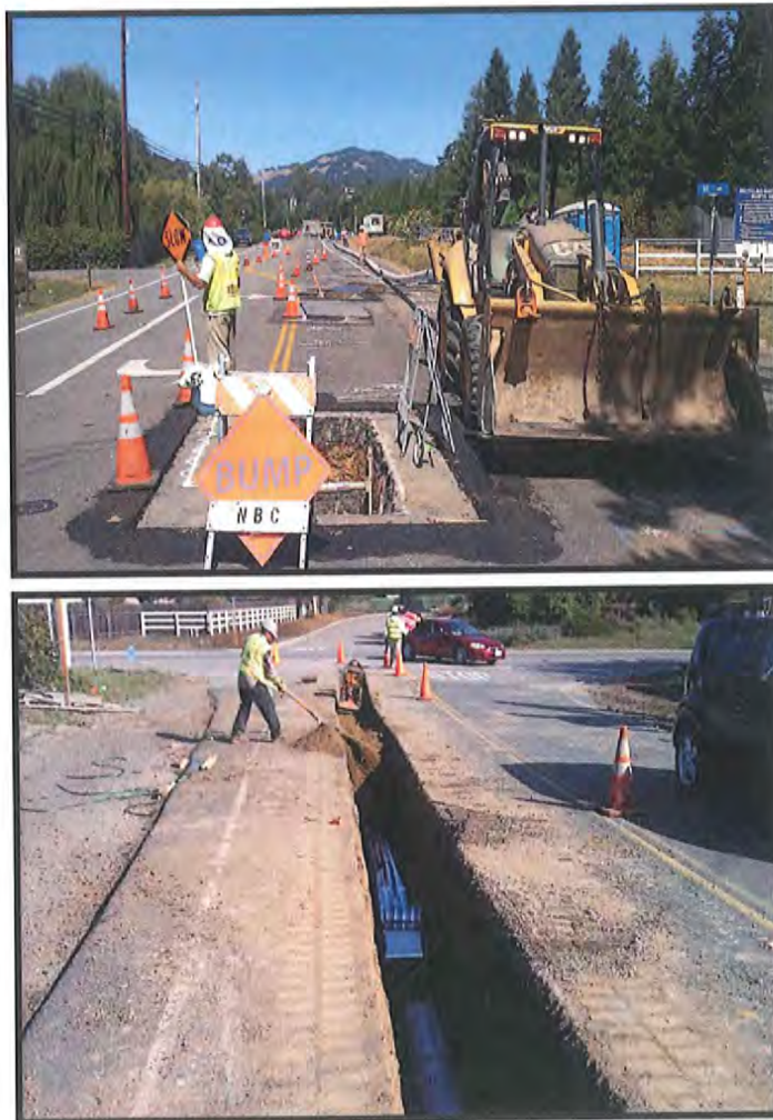
Recycled Water Segment 1 & 3
