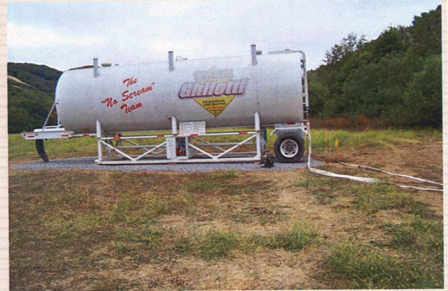
Well Water for Pressure Testing Pipe
