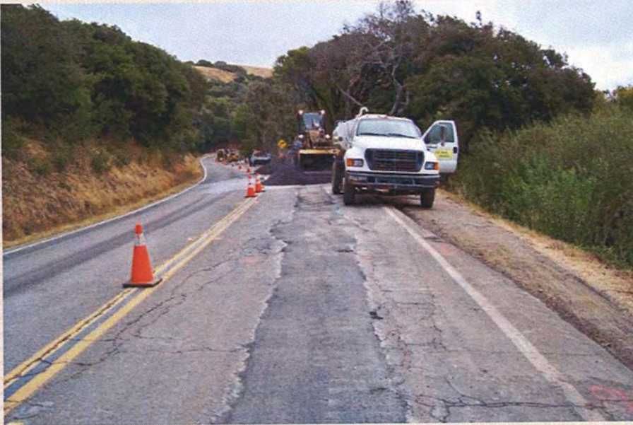
Hot Asphalt Paving same day
