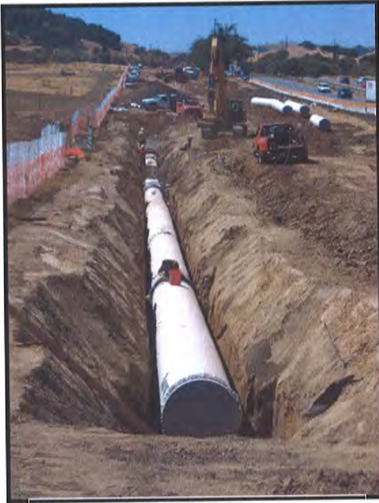
Aqueduct Energy Efficiency Project
