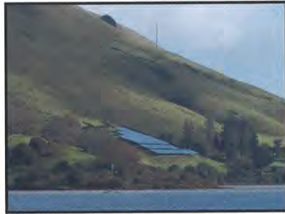
Stafford Lake Solar Power Installation
