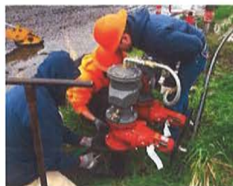
Fire Service Installation at the Redwood Landfill
