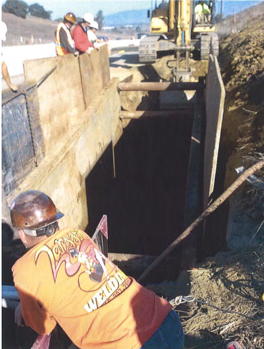
Pipe Excavation in Reach B
