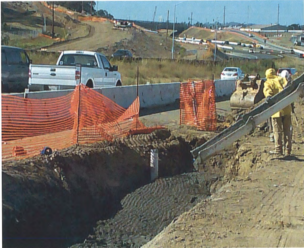
Placement of CDF on Pipeline in Reach A
