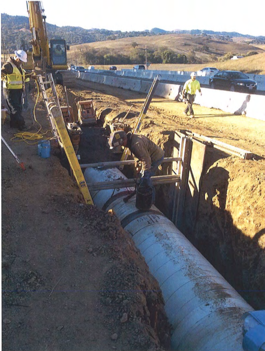
Pipe Installation in Reach B
