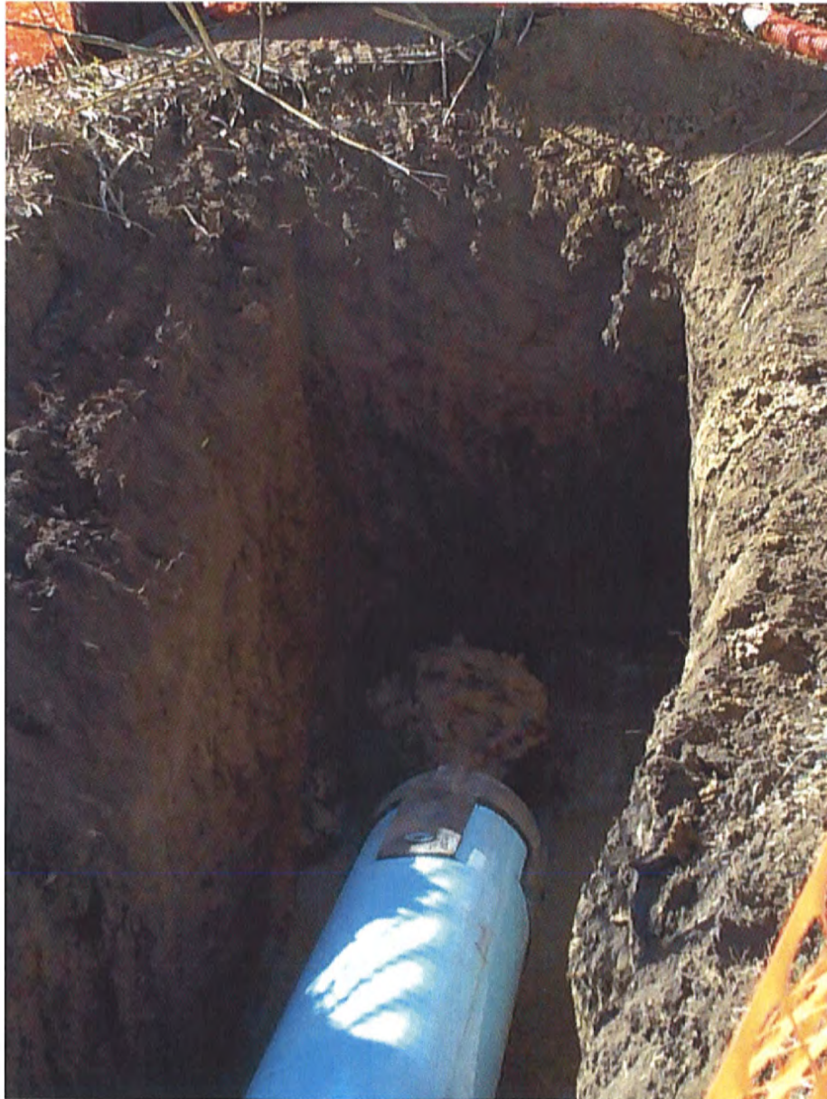
HDD Installation of Pipe (D3)
