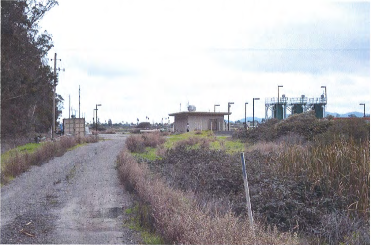
200 feet distance looking south towards hwy 37. Antenna 12 feet above roof.
