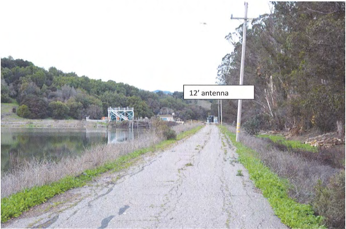
400 feet distance looking north. Hwy 37
