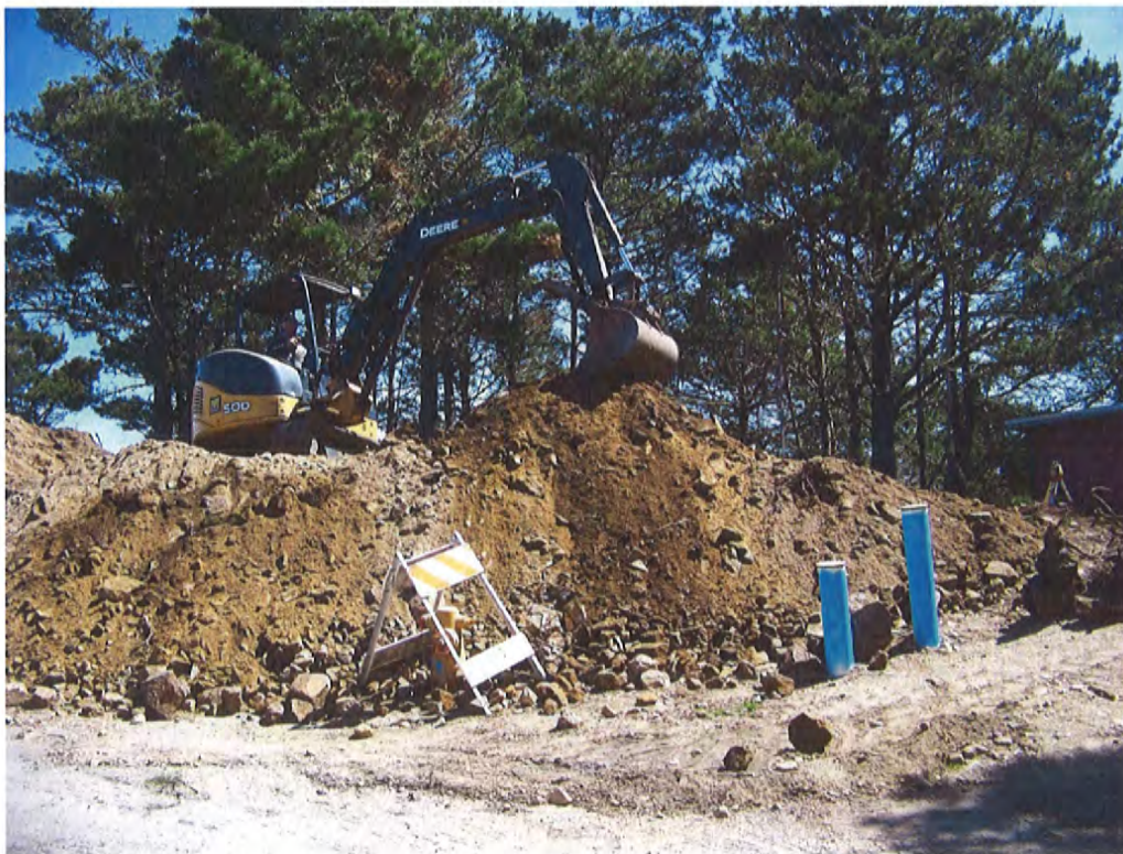
April 22, 2020: View looking North from driveway circle. Valve risers for new isolation valves on left of picture.
