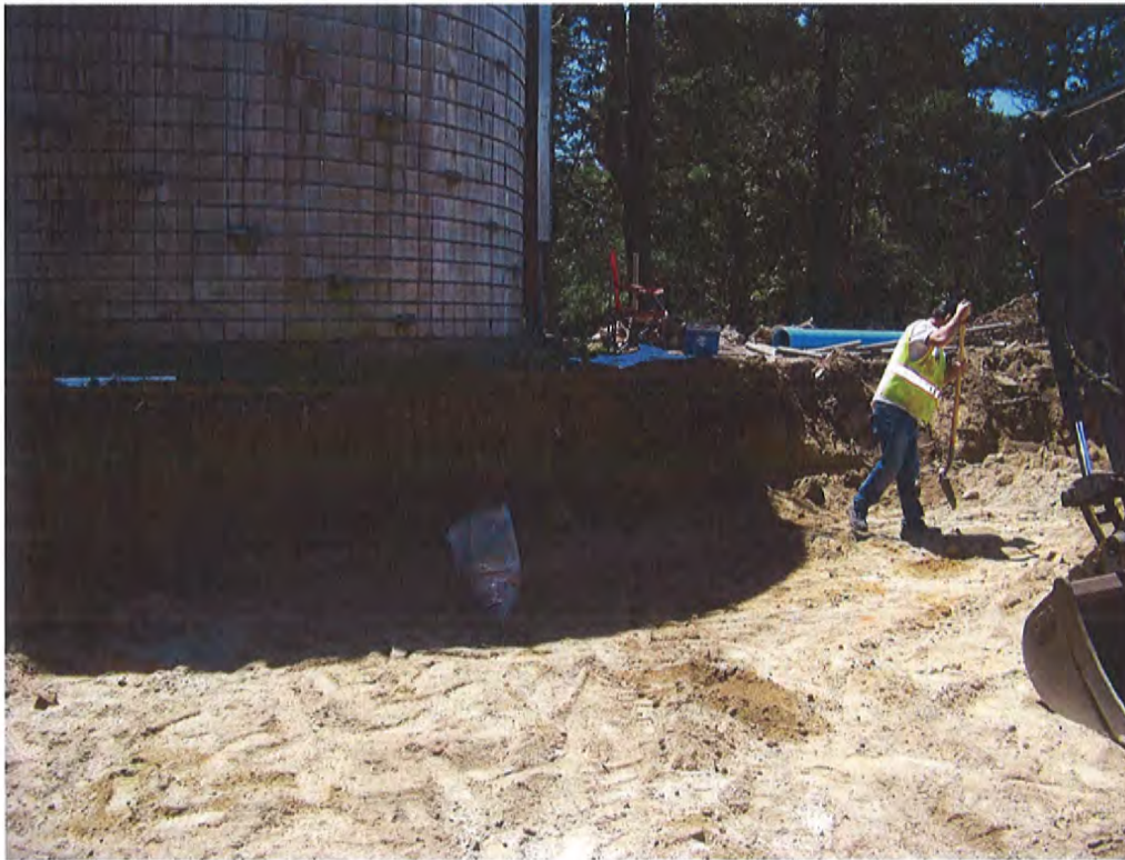
May 4, 2020: Tank subgrade being leveled and compacted. Tank 4B visible on left.
