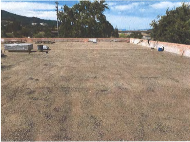
Removal of the rock from existing roof.
