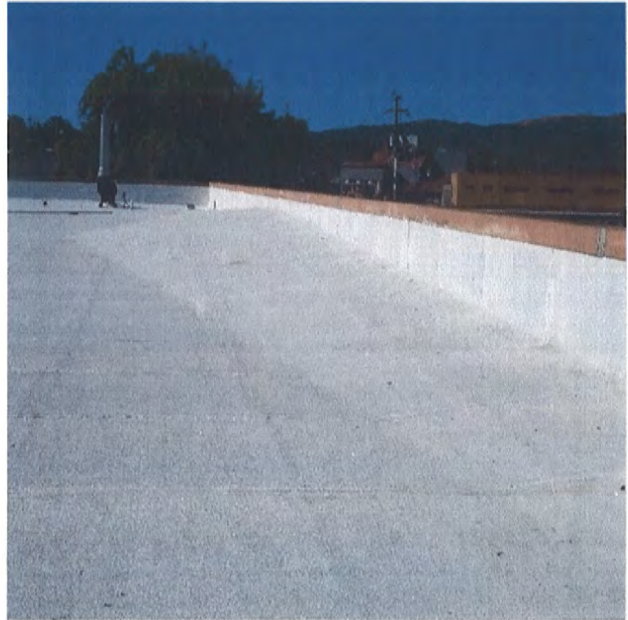
This is the view of the new cricket on the West. Which will eliminate the rain puddling issues we had in the past.
