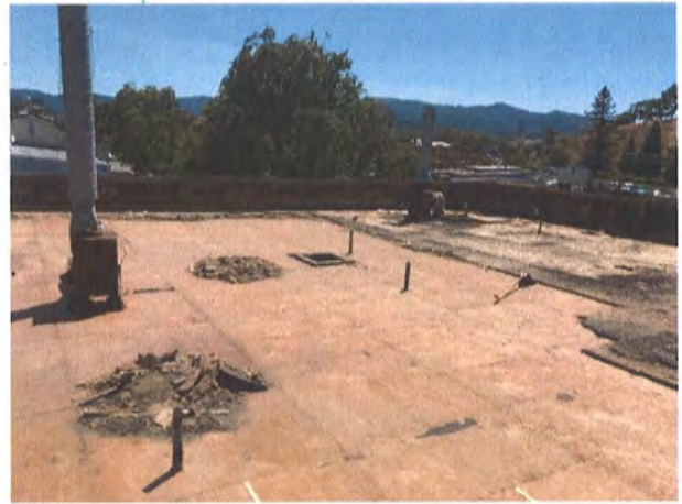
Old roofing materials removed to plywood sub straight.
