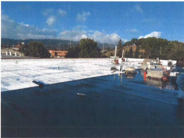
The top layer is a single layer of Polyglass Polyfresko white granular surfaced fire rated white modified bitumen.
