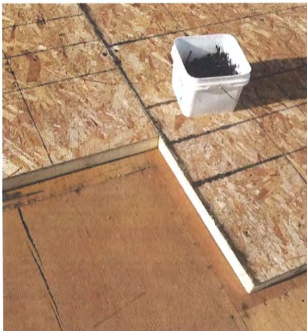
New 2" poly urethane ridge board insulation with a 7/16" OSB board laminated to the top.
