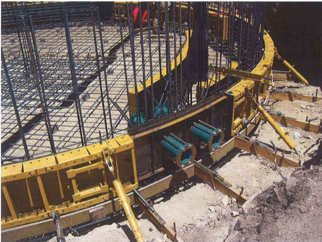
June 18, 2020: Foundation and wall forms being assembled. Inlet and outlet pipes shown.
