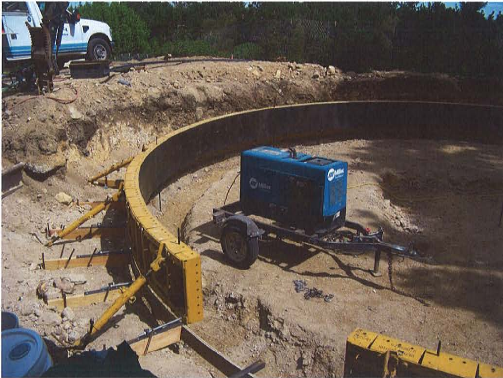
June 10, 2020: Foundation and wall forms being assembled. Looking North from driveway.
