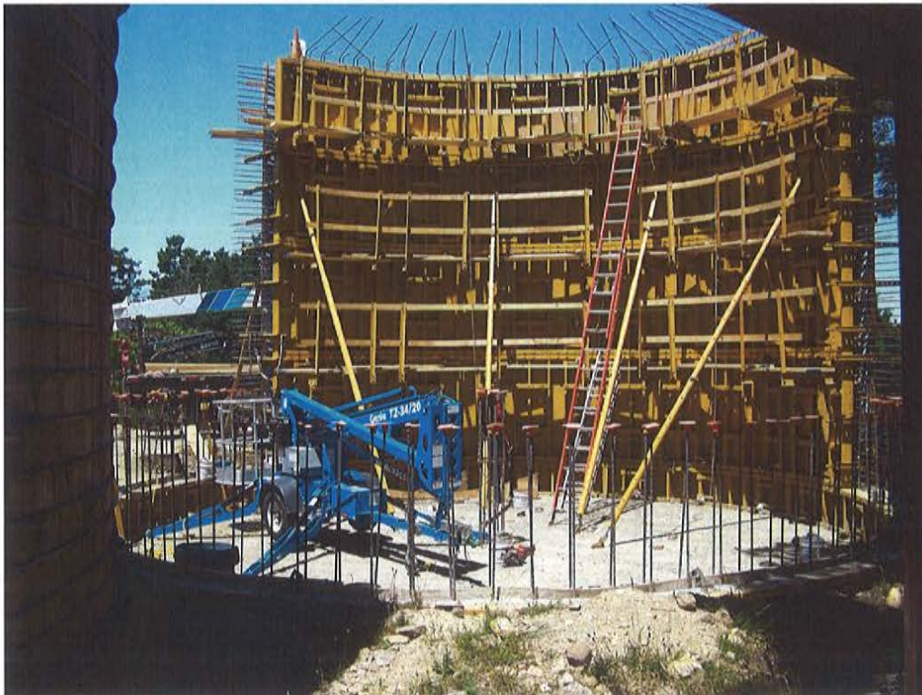
July 28, 2020: First wall segment forms in place, total height 24 feet. Tank 4B visible on left.
