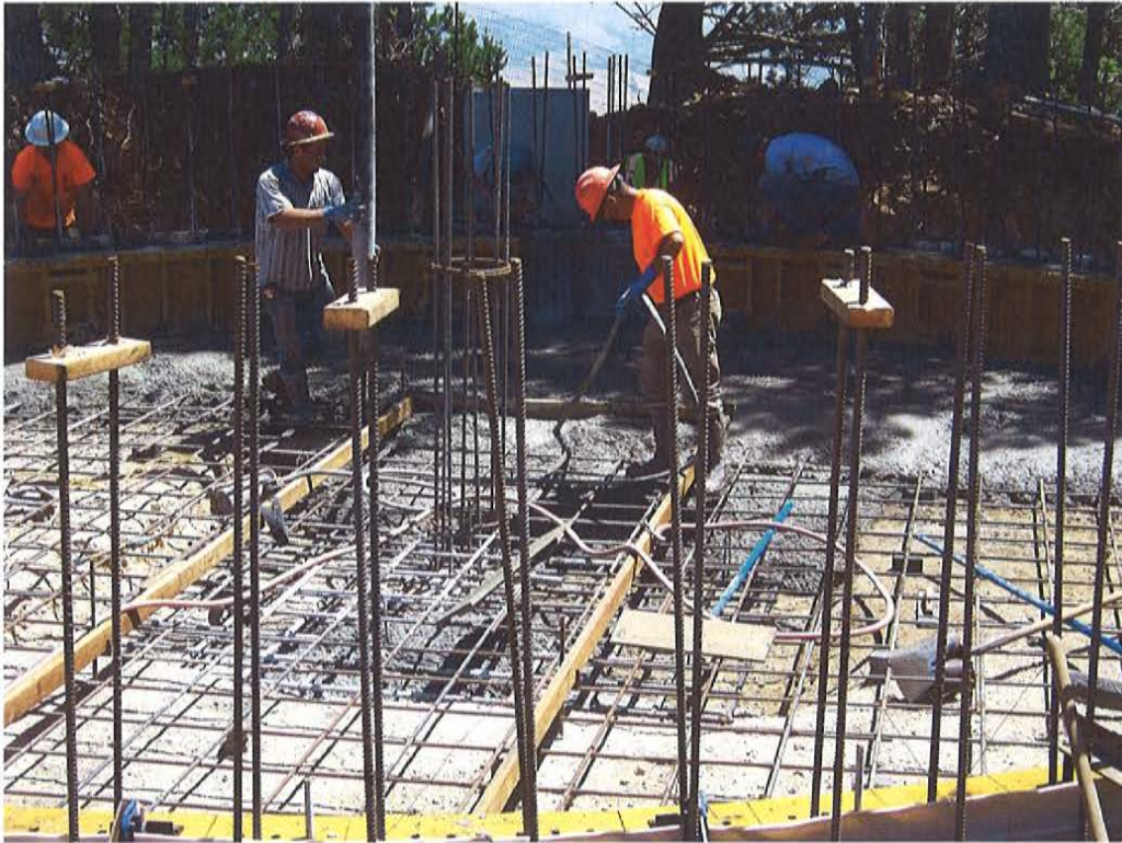
July 1, 2020: First concrete placement, foundation, floor and two feet of shell wall.
