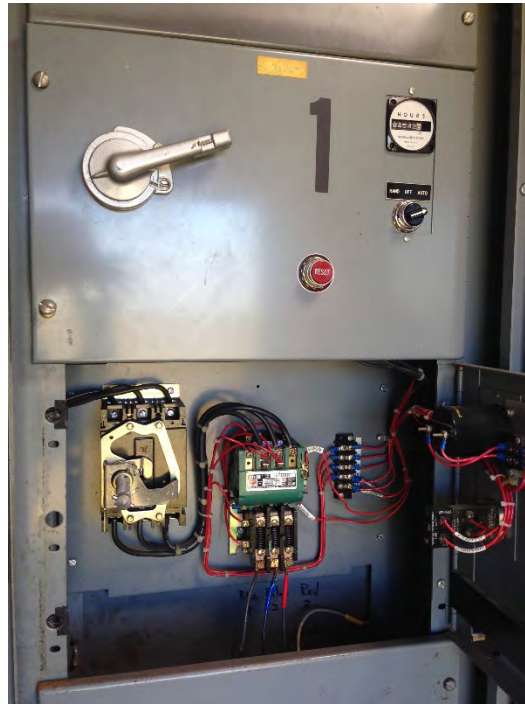
Figure 5: Treatment Ponds Motor Controller Compartment
