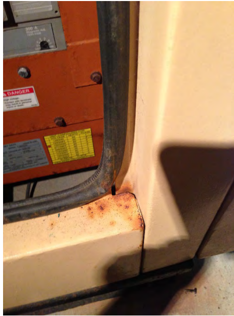
Figure 2: Standby Generator Enclosure Surface Corrosion
