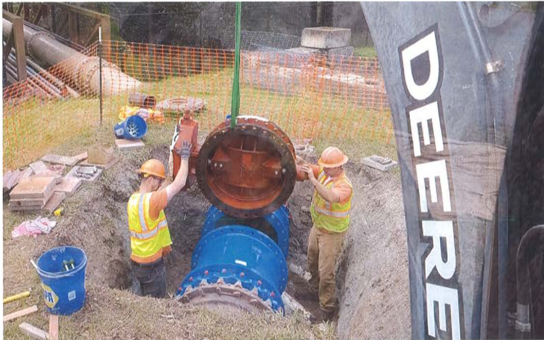
Crews working on Stafford Treatment Plant replacing a failing 30" Butterfly Valve to the Recovery Pond.
