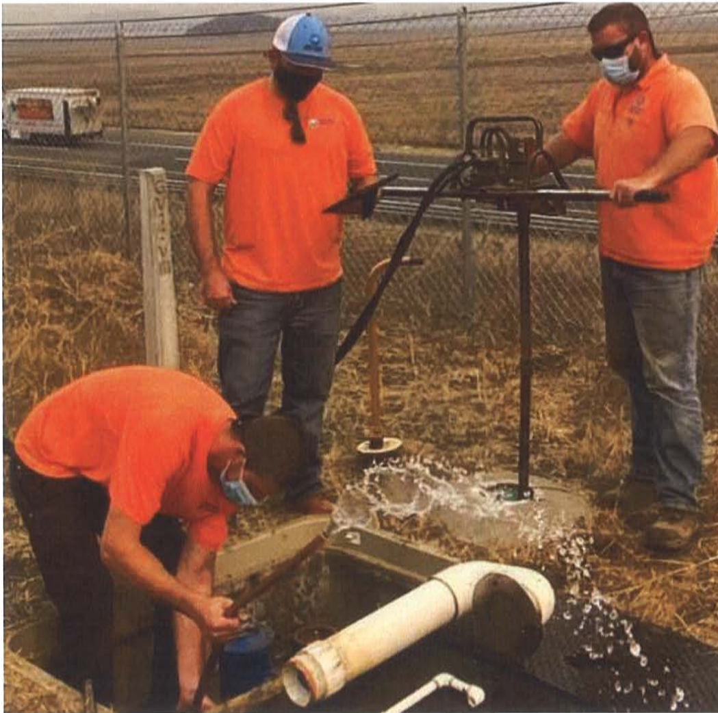
Crew working on air valve testing and repair.
