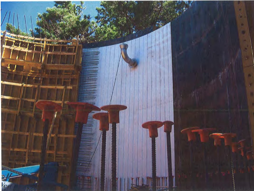
August 13, 2020: Second wall pour forms. Exterior form in place, with overflow pipe and wood patterned form liners.
