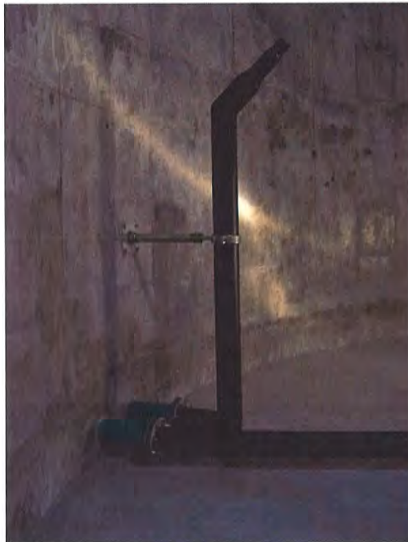
March 15, 2021: Interior piping complete. Inlet pipe discharges to center of tank. Discharge pipe lays on floor.
