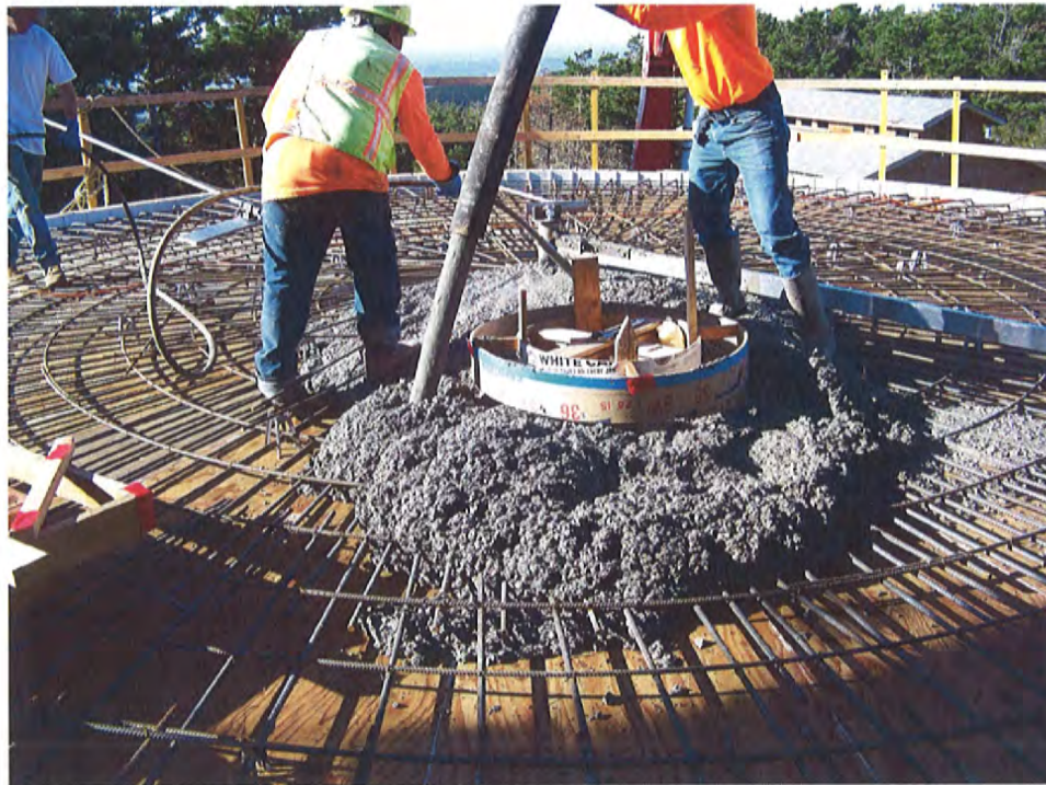
December 29, 2020: Concrete placement of roof. Round forms are for roof vent curb. House at 420 Drakes View Drive is visible in upper right of photo.
