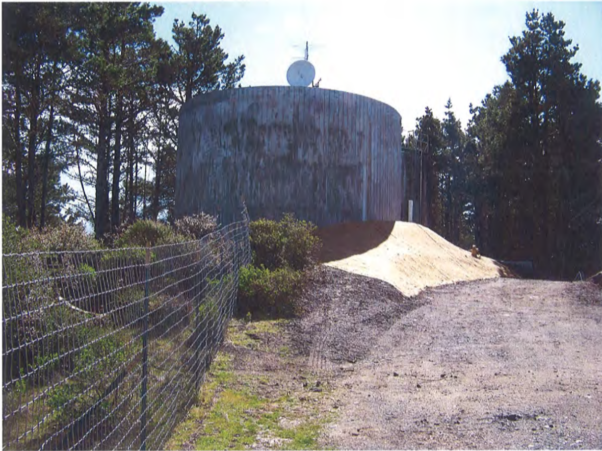
March 10, 2021: View of completed tank and berm from Driveway. Staining of tank is still required. Driveway upgrade and landscaping on berm by District to follow contract completion.
