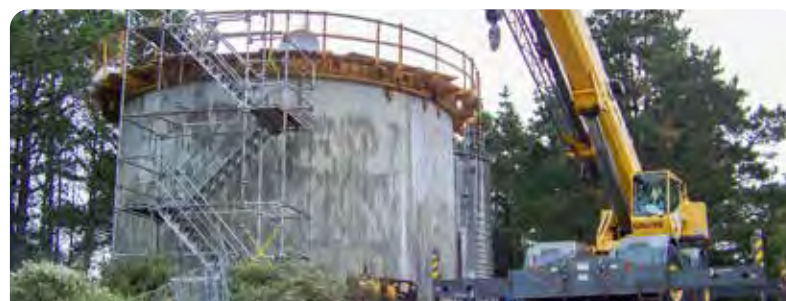
PRE tank 4 construction
