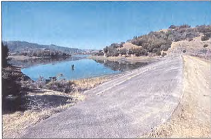
The Stafford Lake dam lines part of the reservoir on Friday in Novato. The lake is the only reservoir in the North Marin Water District.
