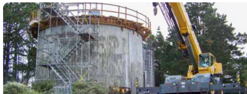
PRE tank 4 construction
