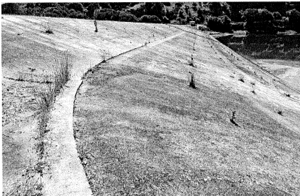
Photo 2: View of the upstream face as seen from the left abutment. Vegetation growing in the cracks needs to be removed.
