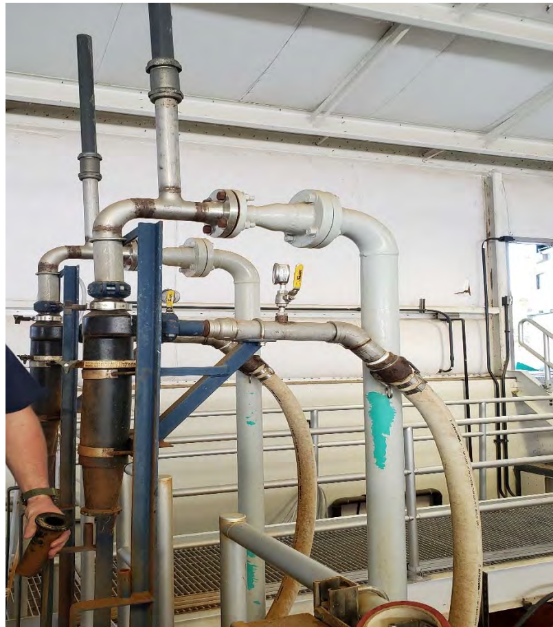
Figure 2. Hydrocyclone Pair on the Deck of an Actifloc Unit
