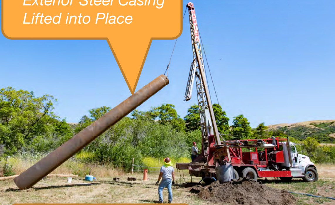
Maggiore Brothers Drilling, Inc. Starting with Bucket Auger Rig
