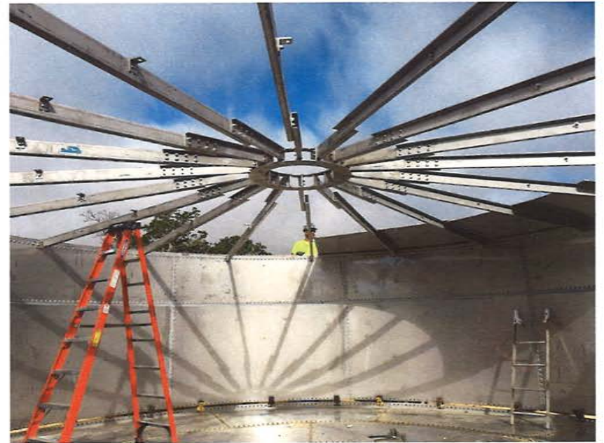
Structural Roof Installation
