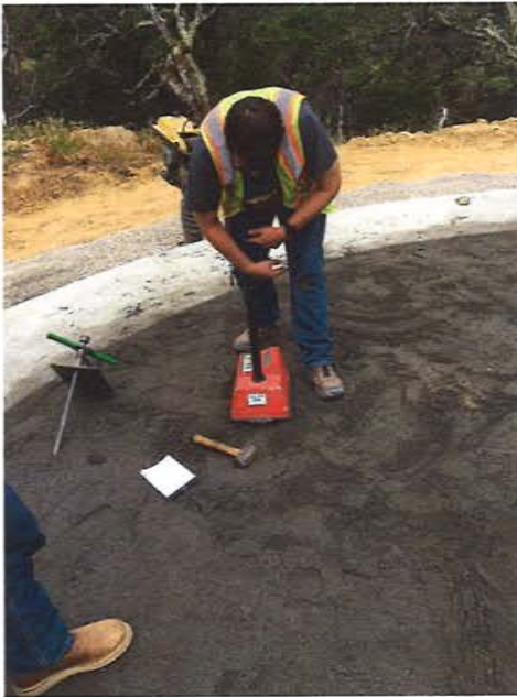
Compaction Testing of Sand Fill
