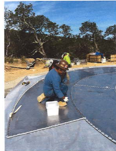
Floor Plate Installation with Sealant
