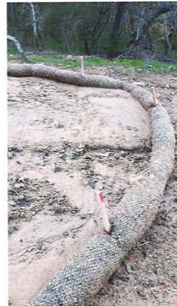
Construction Waddles
