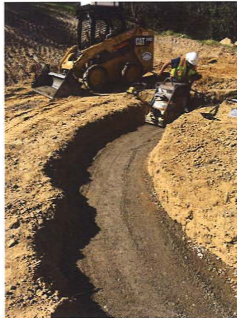
Ring Footing Excavation
