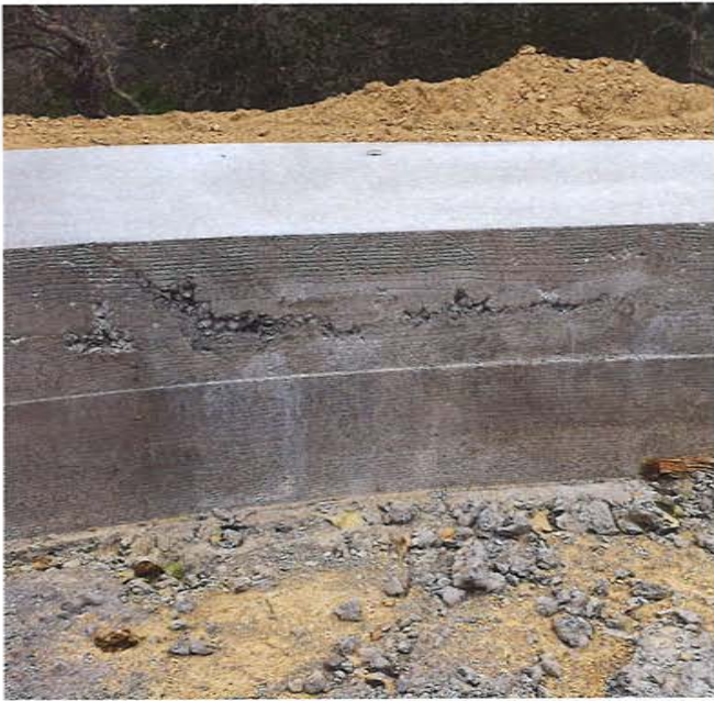
Completed Ring Footing
