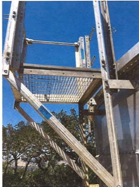
Installation of Appurtenances
