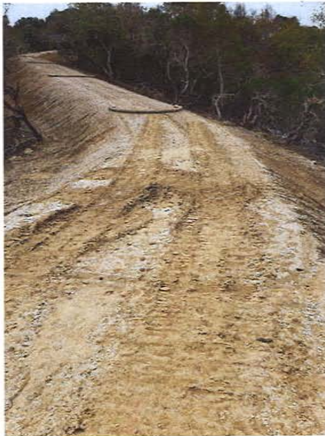
Final Rough Grade Pre-Rain
