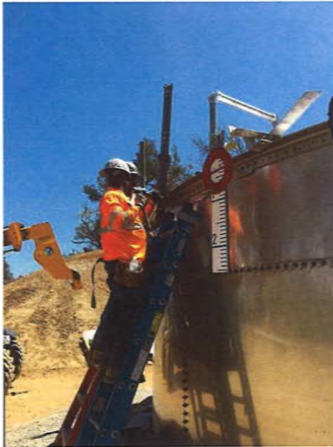
Installation of Appurtenances
