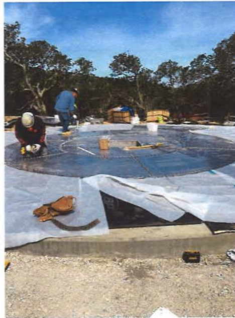
Tank Shell Floor
