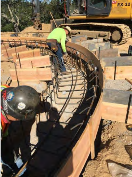
Rebar Placement
