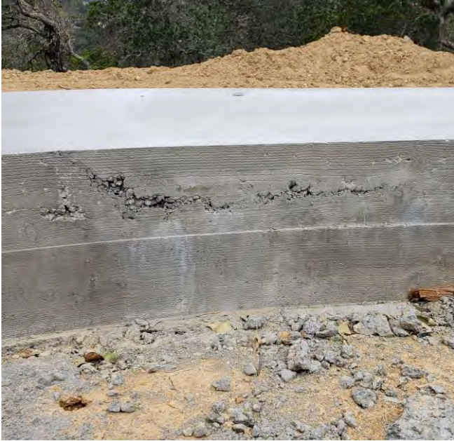
Completed Ring Footing
