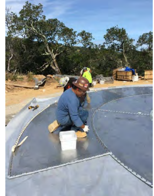
Floor Plate Installation with Sealant
