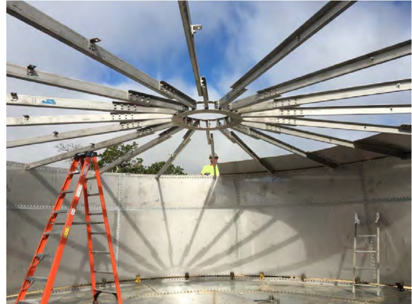
Structural Roof Installation
