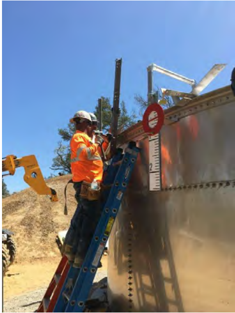
Installation of Appurtenances
