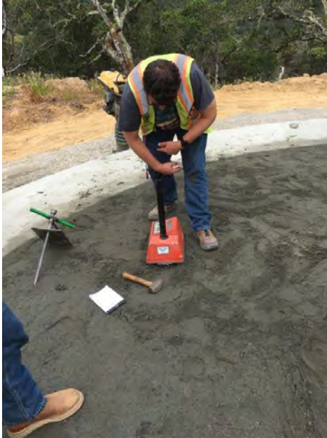
Compaction Testing of Sand Fill
