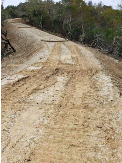
Final Rough Grade Pre-Rain
