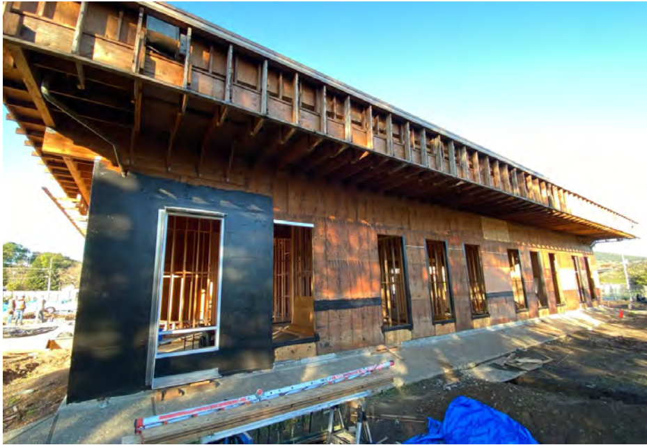
Soffit Framing Begins
