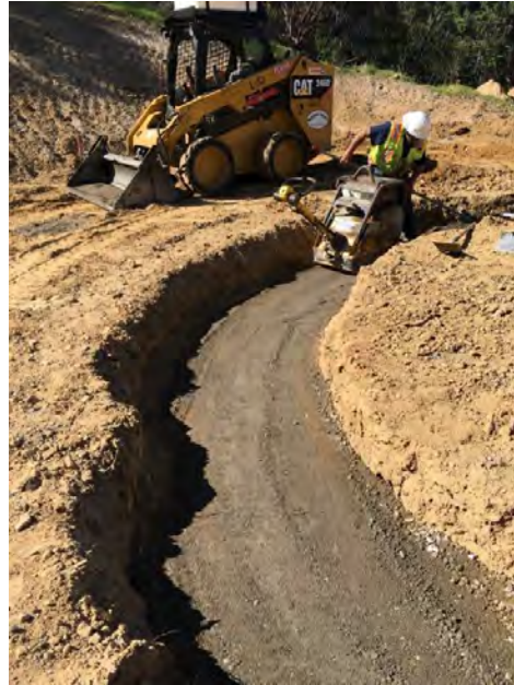
Ring Footing Excavation
