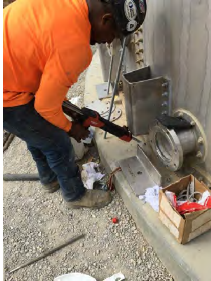
Epoxy Dowel Install
