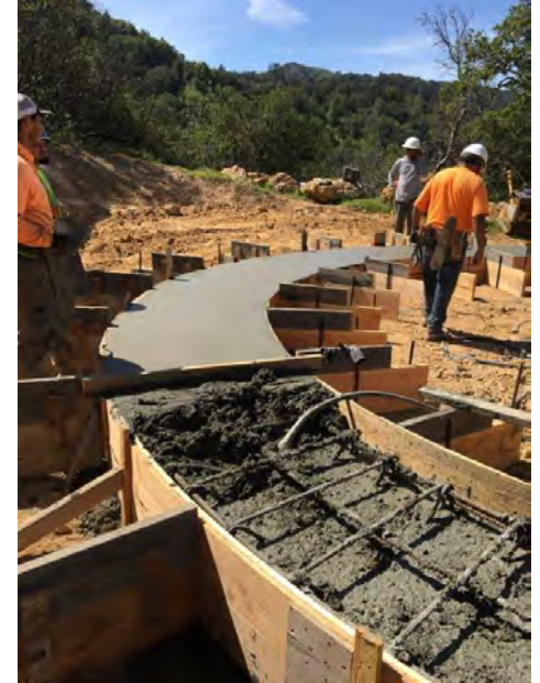
Concrete Finishing
