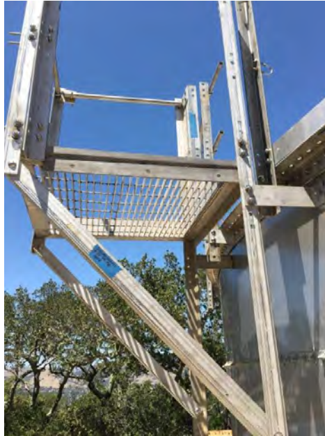
Installation of Appurtenances
