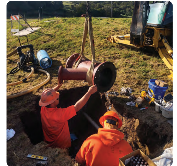
Crew installing a tee for Gallagher Well Project in West Marin
