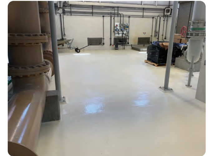
STP - Coat top of concrete clearwells
