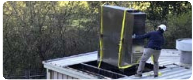
Stafford Treatment Plant High-Service Pump Station variable frequency drive replacement.
