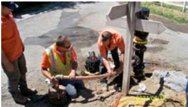
Replacing 6" AC Pipe - Glen Rd
