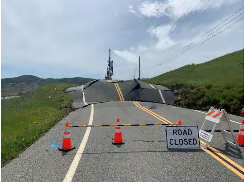
Looking north along pipeline alignment
