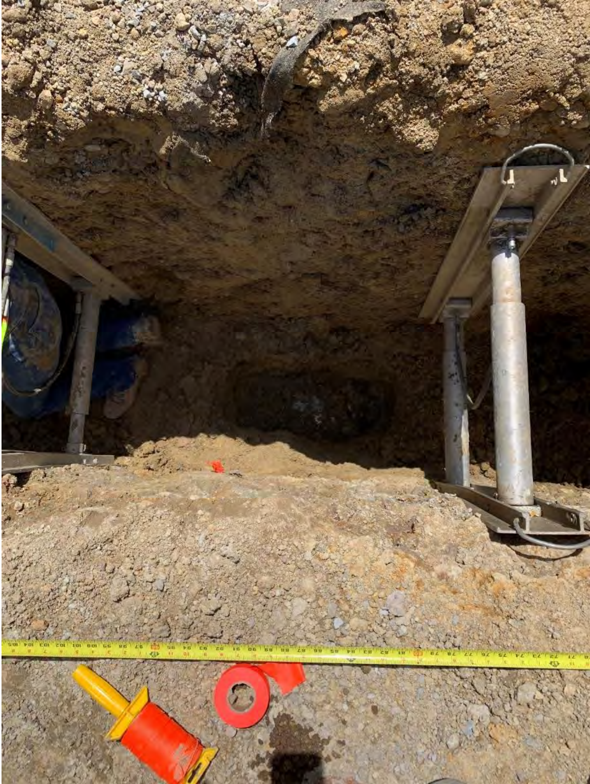
Test Pit #2 (top of pipe exposed)
