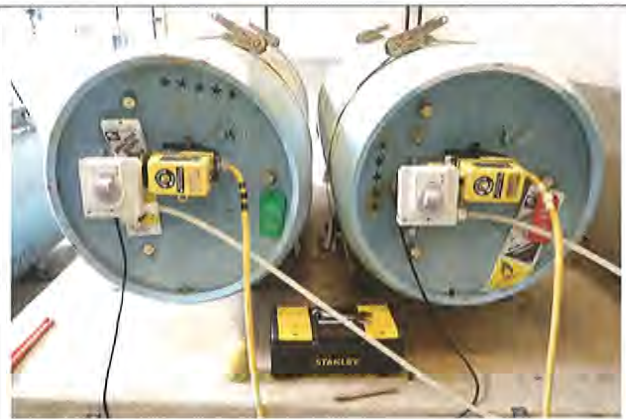
Excerpt from Photograph 19 showing transparent chlorine vacuum tubing, vacuum regulator, and emergency shut off valve on each one-ton container.
