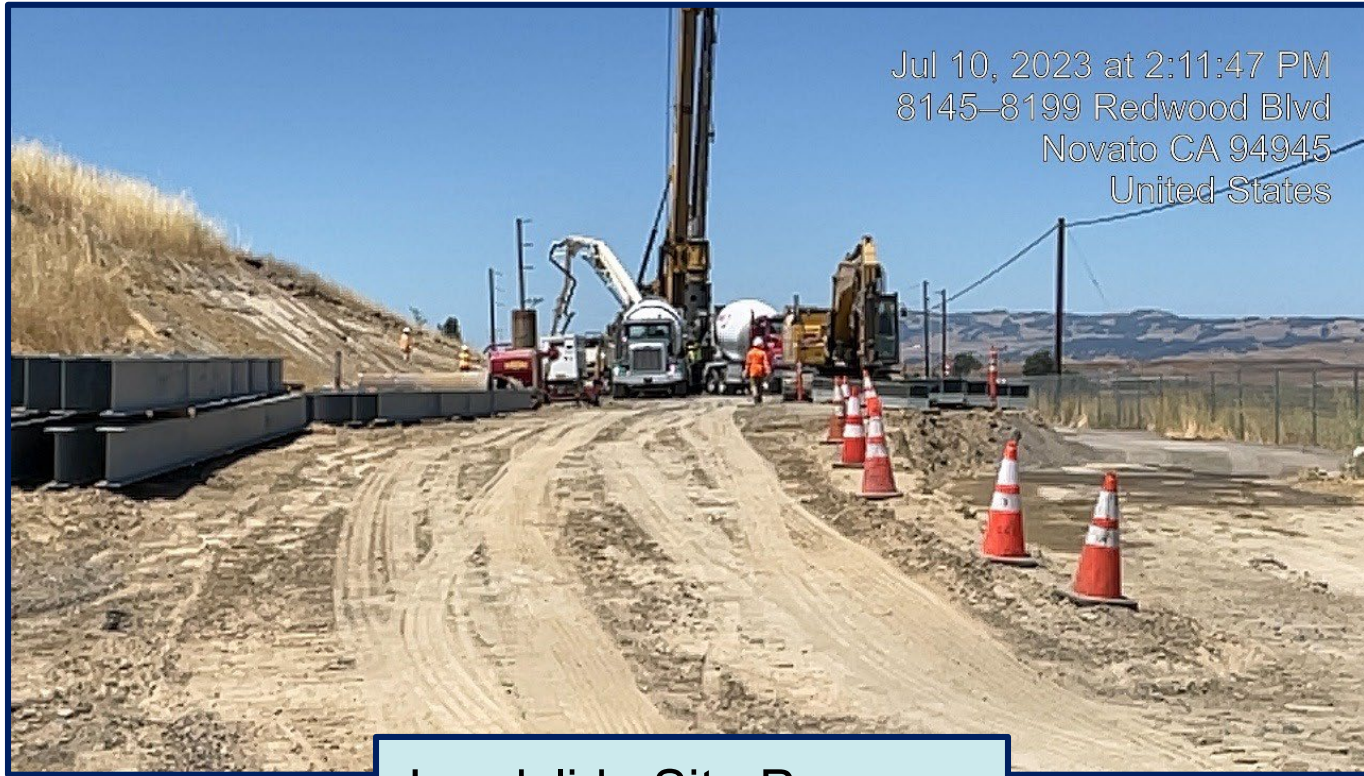
Landslide Site Progress
