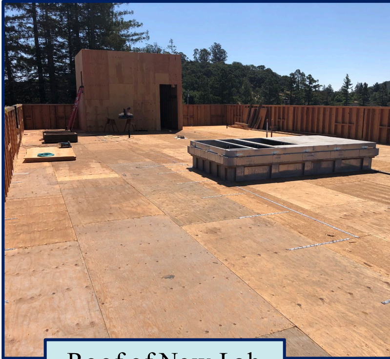
Roof of New Lab
