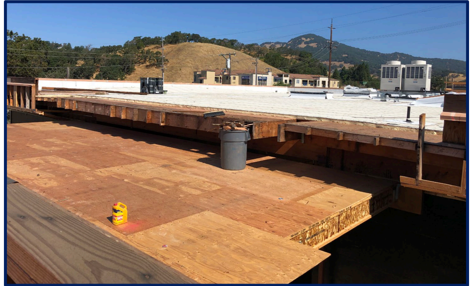
Roof of Staff Lunchroom
