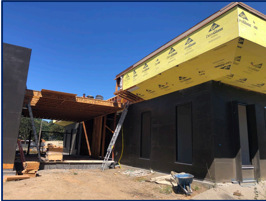
Soffit Sheathing
