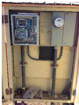
Figure 4: North Street Lift Station Level Controller and PG&E Meter
