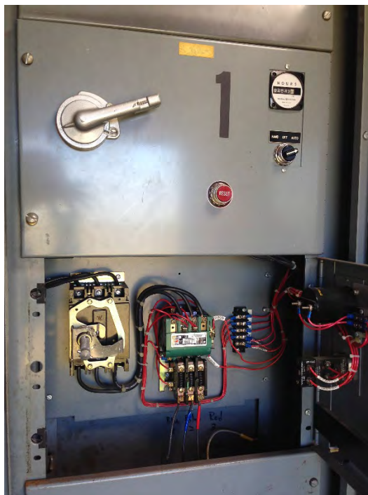
Figure 5: Treatment Ponds Motor Controller Compartment
