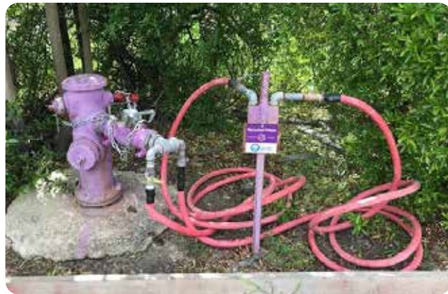
Novato residential recycled water fill station.
