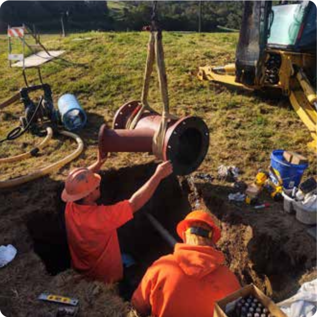
Crew installing a tee for Gallagher Well Project in West Marin
