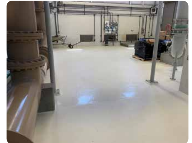
STP - Coat top of concrete clearwells
