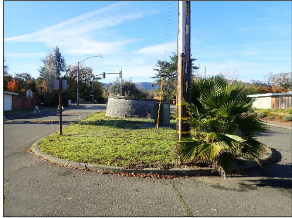
Photo of the Existing PS Site.
