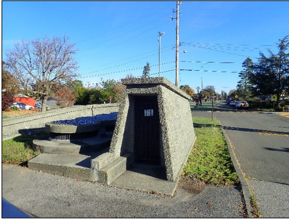
Photo of the Existing PS Site.
