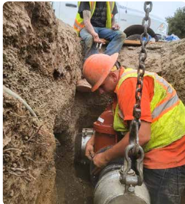
Crews installing tapping machine for an 8 inch tap.
