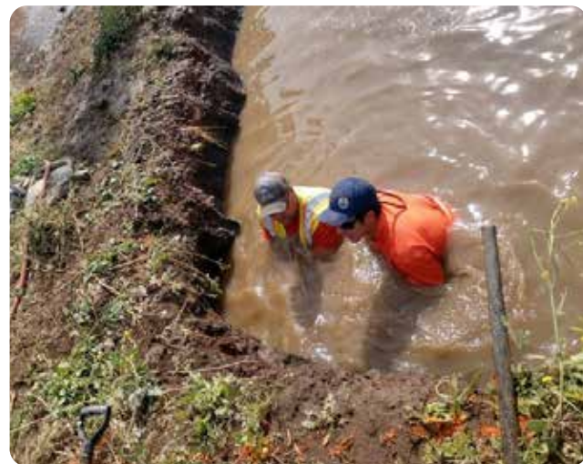
Crews repairing 8 inch water main break.
