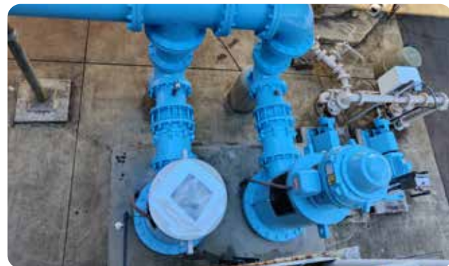
Stafford Treatment Plant - Pipe gallery re-coat.
