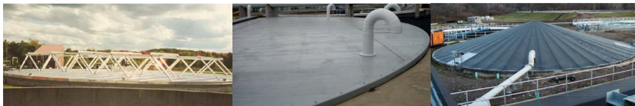
Figure 3-3: From Left to Right – Example Aluminum, FRP and Geomembrane Covers
