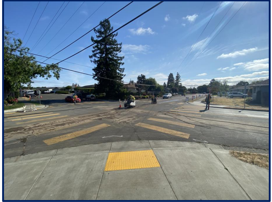
Saw Cutting The Trenches
