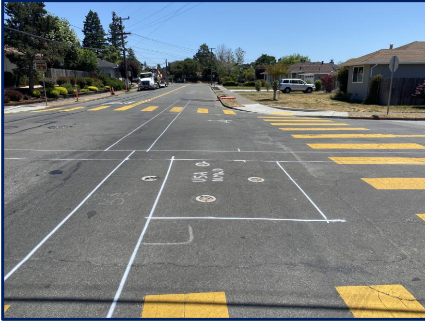
Marking Out The New Alignment
