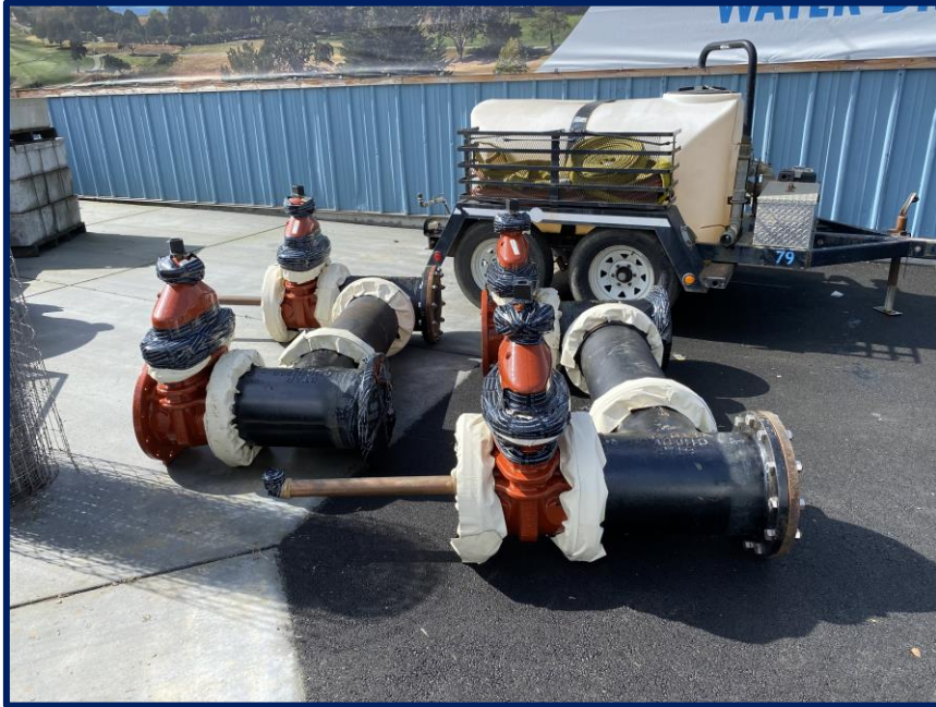
12" Cut-In Valve Assembly Pre-Assembled
