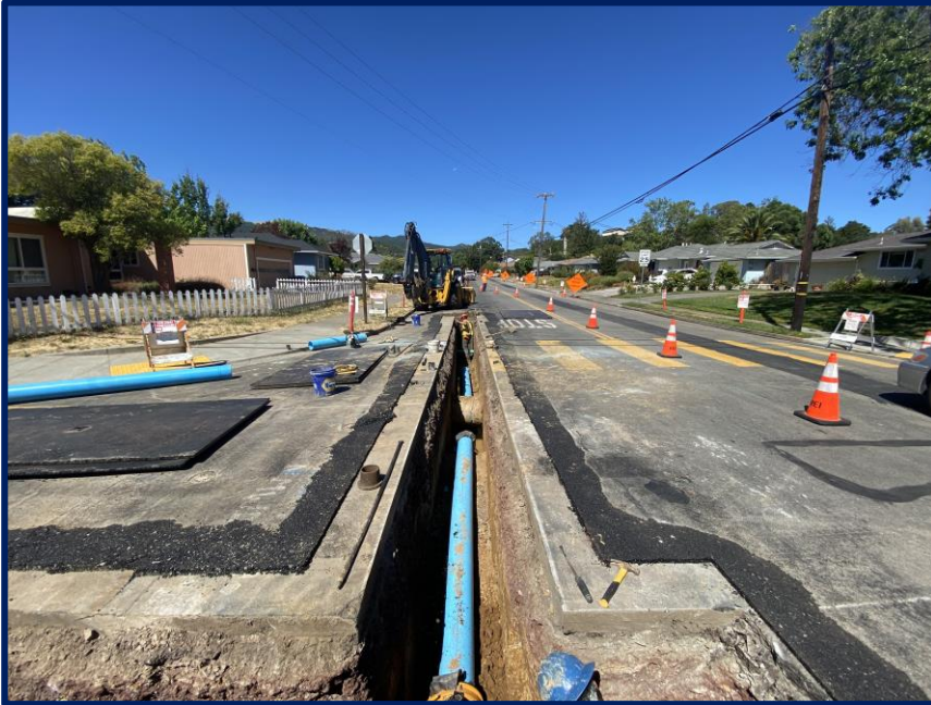
Installing 8" PVC on Cambridge St.
