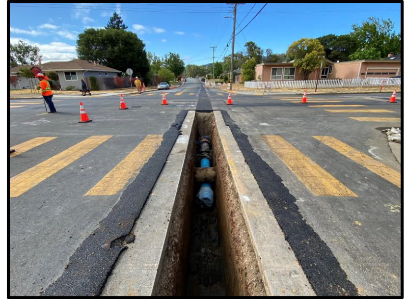
12" PVC Over Sewer, Under Storm Drain, Under Gas, and Match Existing Water Grade for Tie-In
