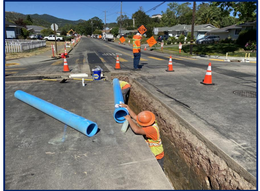
Disinfecting PVC Main With Chlorine
