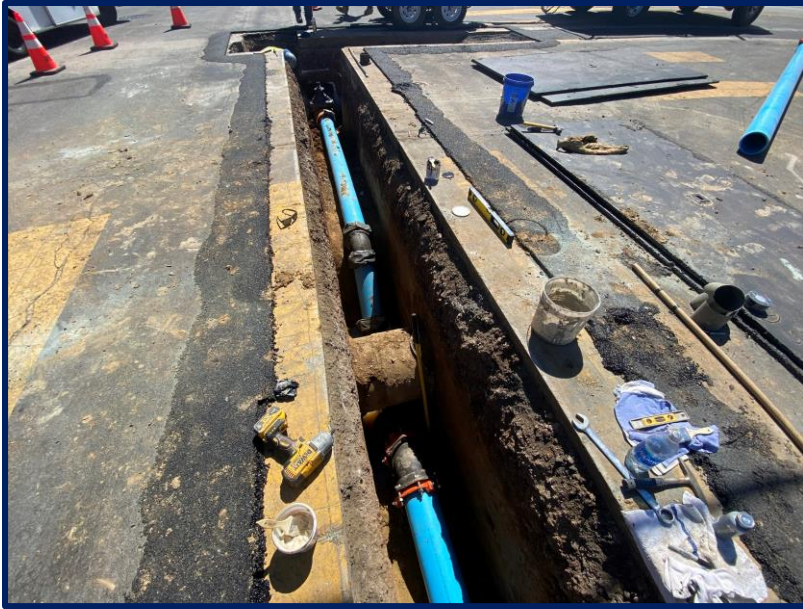
Installing 8" 45 Deg Elbows for Existing Storm Drain
