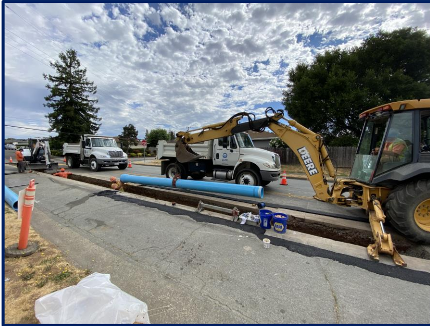
Lowering 12" PVC In Trench
