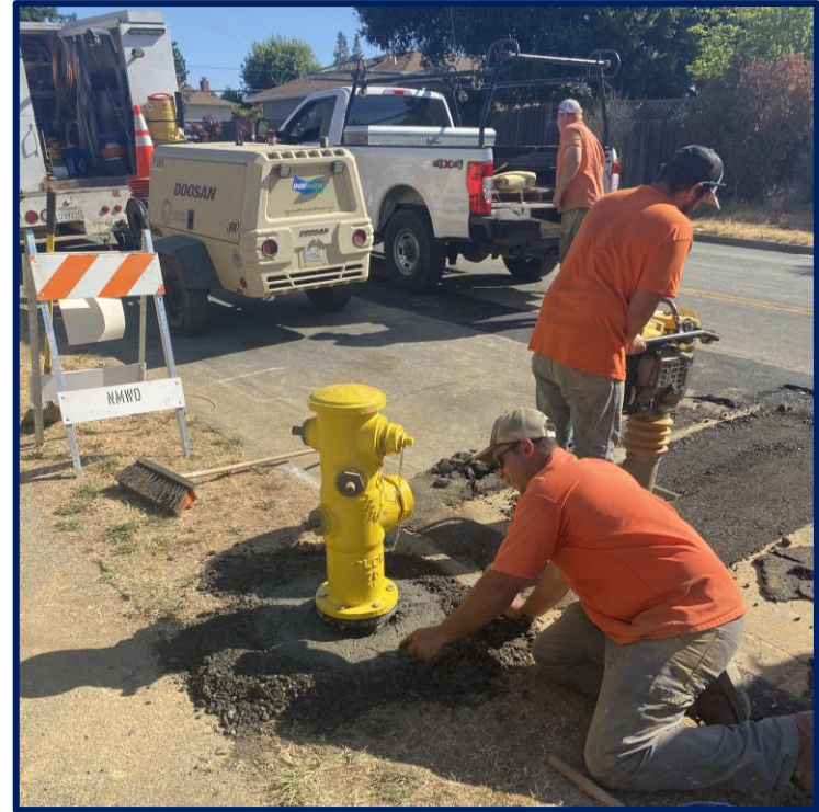
New Hydrant with 6" Hydrant Main
