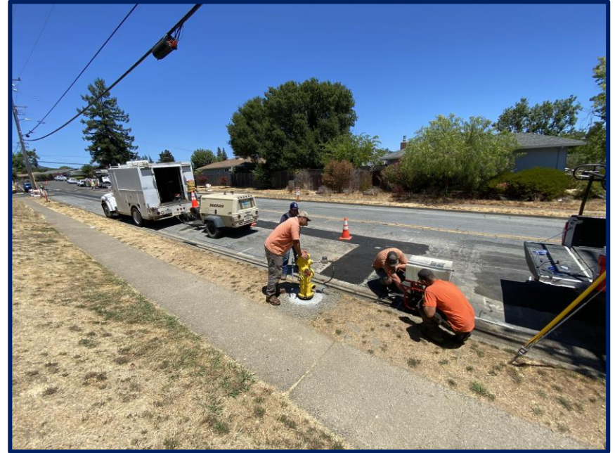
Pressure Testing New Water Main
