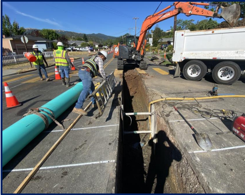
Abandoning Existing Water Main for New Sewer Main
