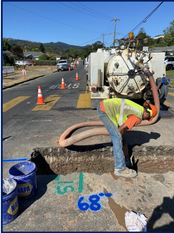
Potholing Existing Sewer and Water
