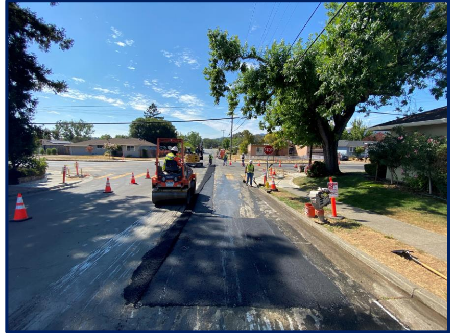
After 8" Asphalt Plug
