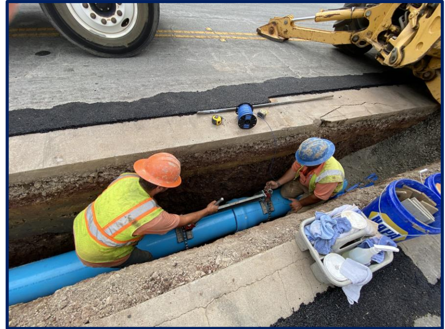
Inserting 12" PVC Bell and Spigot
