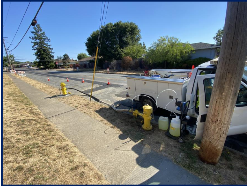
Chlorinating New Water Main
