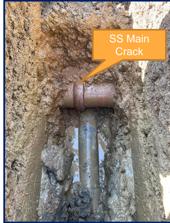
Sewer Cracked Above the Water Main
