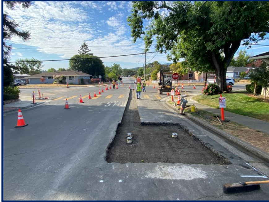
Before 8" Asphalt Plug
